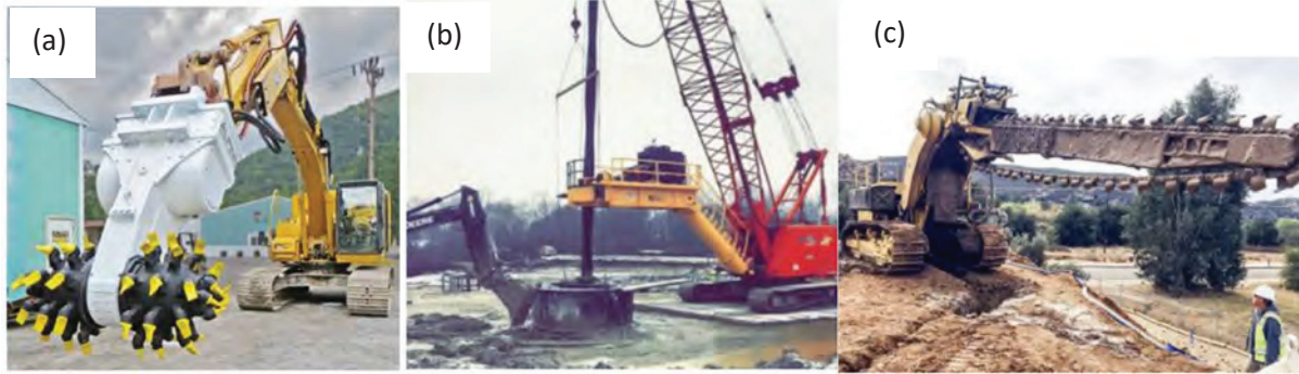
Figure 2. In Situ Soil Mixing. (a) Equipment used to mix to a depth of 25 ft (Source: Redox Tech), (b) Deep soil mixing where blending can be completed to 90 ft depth (Source: GeoSolutions) and (c) Trenching technique used to either blend or create a PRB trench to a nominal depth of 25 ft bgs (Source: GeoSolutions).
