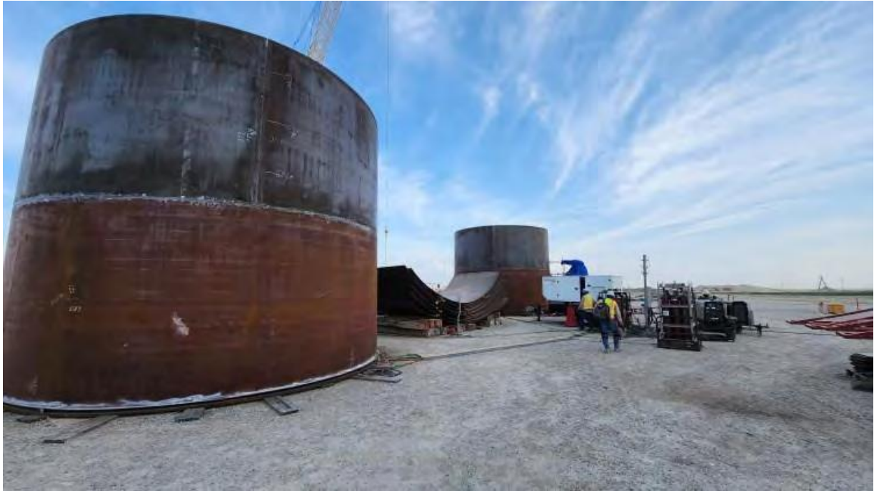
Photo 3: Amine Tank Fabrication (Laydown Yard)
