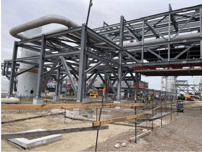
Photo 3: 311R02 & R03 Train 1 Liquefaction Piperack
