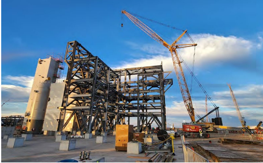
Photo 5: 322A01 Train 2 Cryo Piperack Steel Erection
