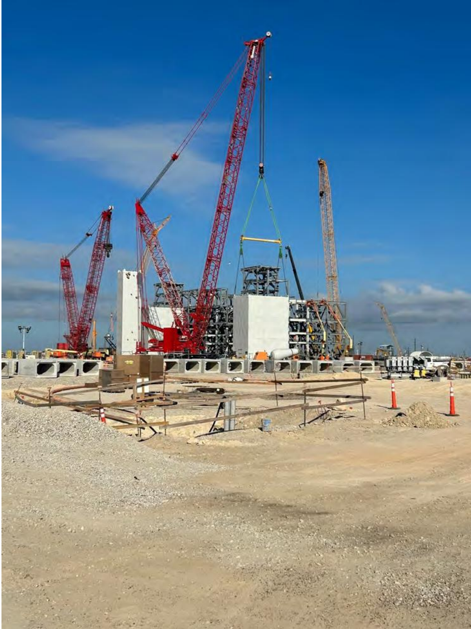
Photo 4: Train 1, Third Cold Box Installation
