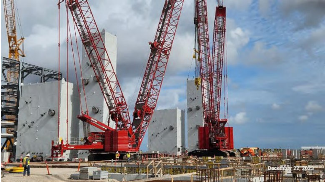
Photo 3: Area 322A03 Train 2 Cold Box Set
