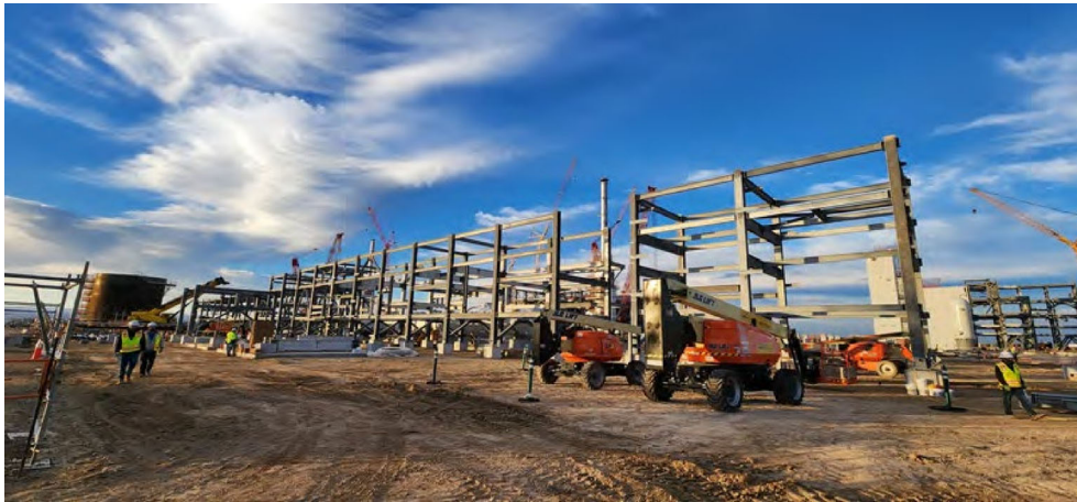
Photo 6: 310R01 OSBL East Piperack Steel Erection
