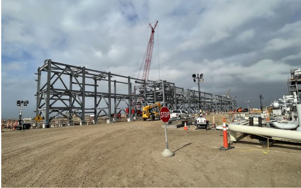
Photo 5: Area 310R08 OSBL West Piperack Erection
