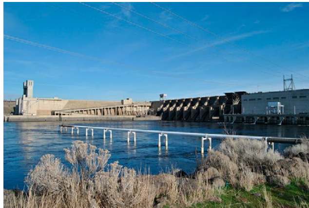
Ice Harbor Dam in Washington uses a run-of-river system, which requires little water storage. Photo from Sarah Wagoner, U.S. Department of Energy's Make a Splash Photo Contest
