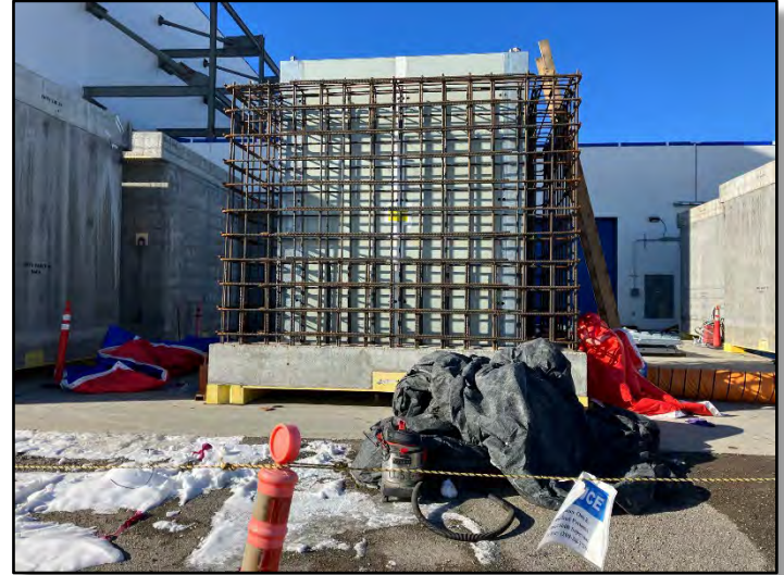
New canister vault construction
