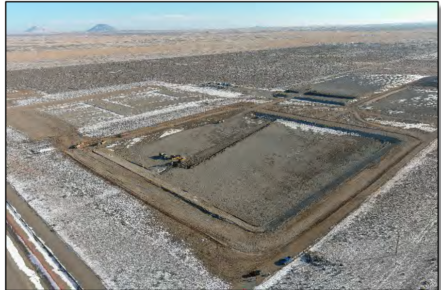
ICDF additional cell and evaporation pond preparation
