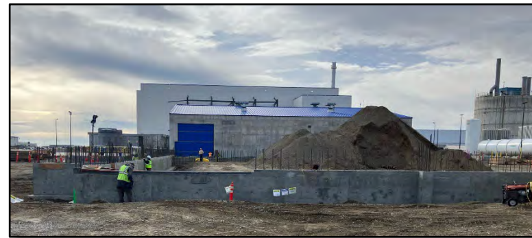
Product Storage Building II stem wall construction
