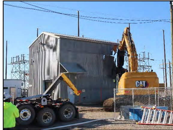
A1W support building demolition before (above) and after (right)
