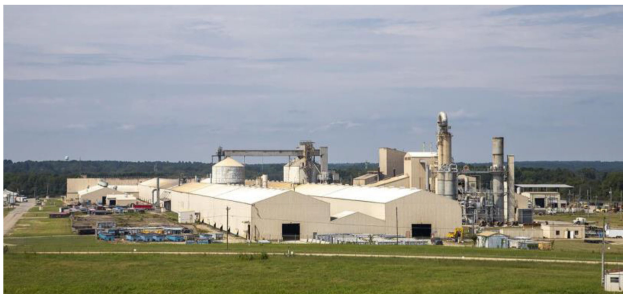
Figure 2-11 Veolia Gum Springs Facility in Clark County, Arkansas
