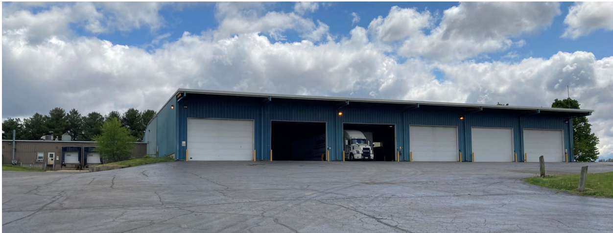
Figure 2-14 CSB-2 (foreground) and CSB-1 (rear left) at the Clean Harbors Pecatonica Site
