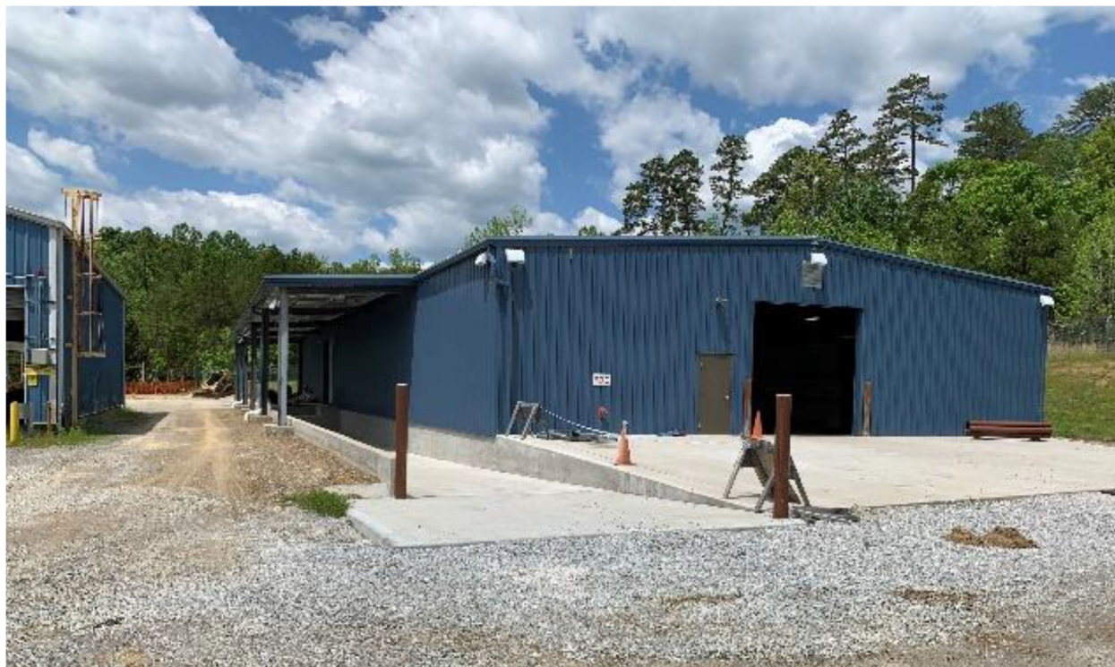
Figure 2-10 Perma-Fix DSSI CSBU
