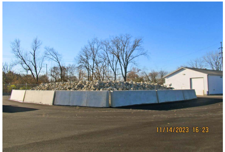
The entombment sits below grade, fully enclosed in a 10-foot-thick concrete barrier. The surface includes a vegetation barrier and loose stone cover, known as riprap, secured by heavy-duty jersey barriers. The city can use the surrounding parking lot as a laydown area.
