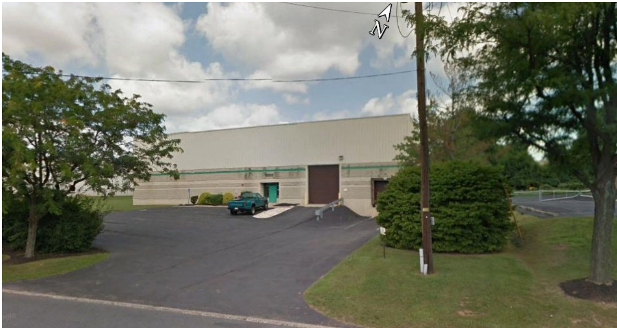
Figure S-8 Bethlehem Apparatus Building 1055
