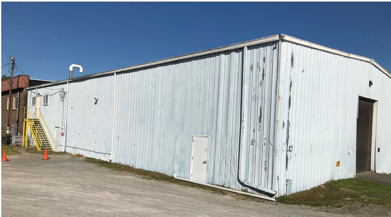
Figure S-13 Storage Warehouse Building at the Clean Harbors Greenbrier Site
