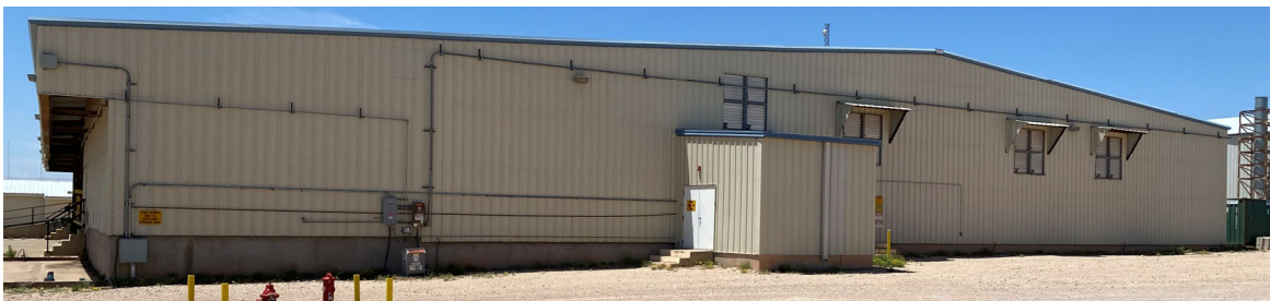
Figure S-5 Container Storage Building at Waste Control Specialists Site
