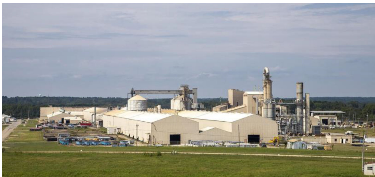
Figure S-11 Veolia Gum Springs Facility in Clark County, Arkansas
