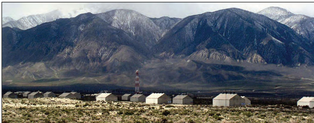
Figure S-3 Existing Storage Buildings at the HWAD in Nevada
