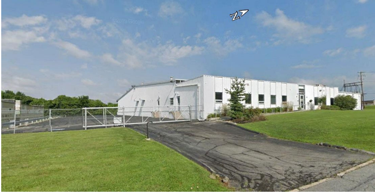
Figure S-7 Bethlehem Apparatus Building 945 (foreground) and Building 935 (rear left)
