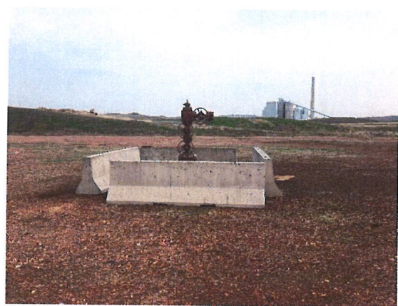
Existing injection well and DFS.
