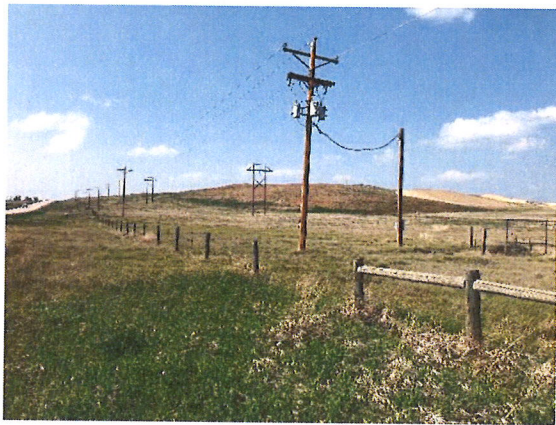
Siting of future injection well site.
