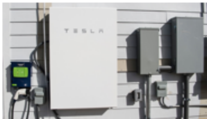
Figure 1. This photograph shows the Tesla PowerWall 2.0 which is the subject of the assessment.
