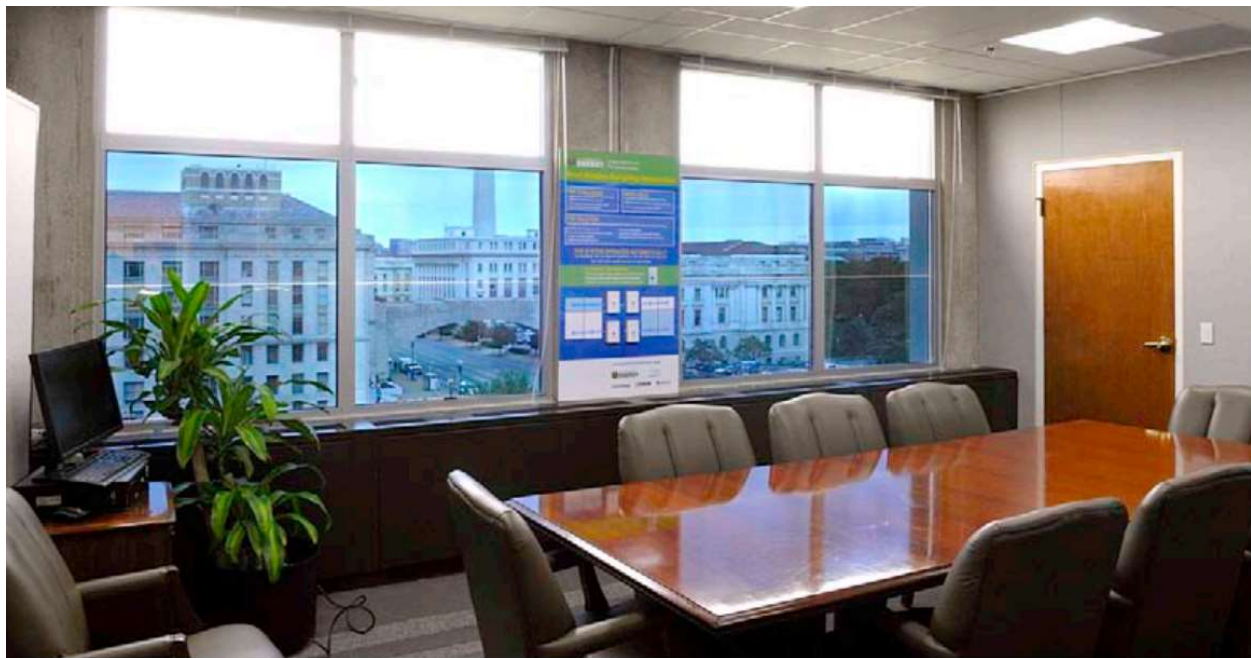
Figure 4. EC windows installed in a conference room in the U.S. Department of Energy Headquarters in Washington DC. Photo courtesy of DOE Photography.
