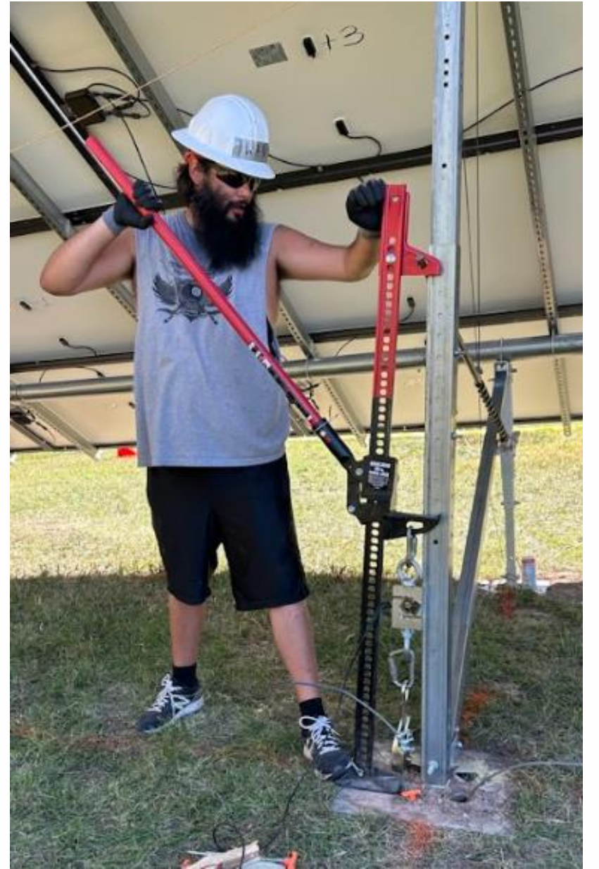
Load test anchor
