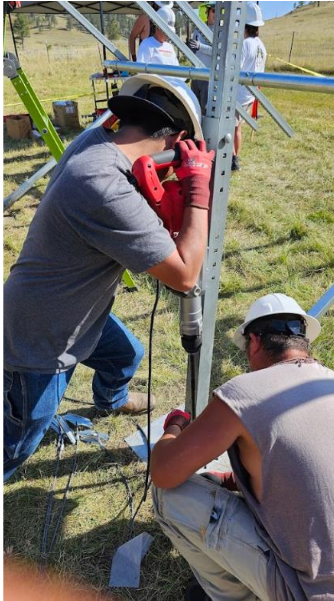
Anchor installation
