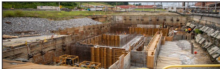
Construction progressing on the headworks facility.
