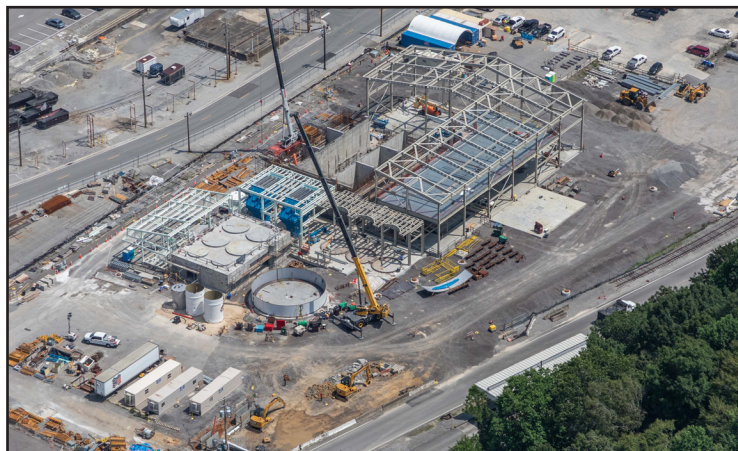
Construction progressing on the treatment plant
