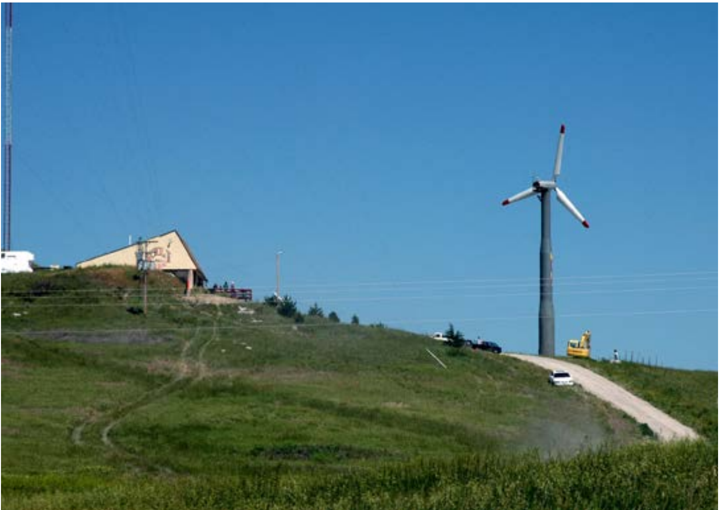
The Lakota Nation installed a 65-kW Nordtank turbine that annually supplies 120 MWh of power to KILI, the Pine Ridge Reservation radio station known as the voice of the Lakota Nation in South Dakota. Photo by Bob Gough, NREL 16258
