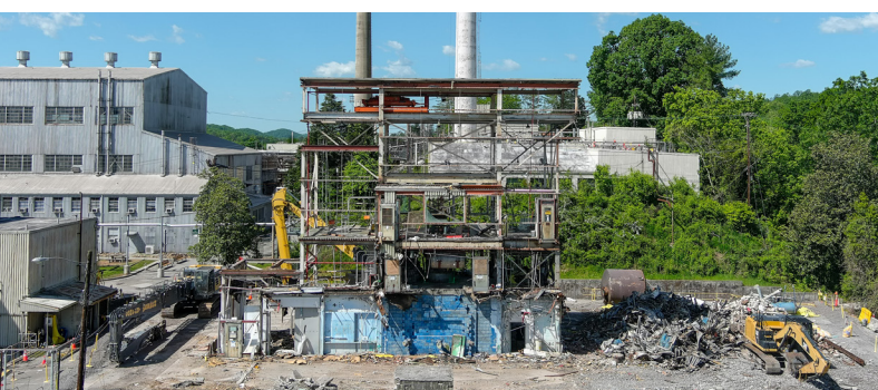
Crews safely take down the Low Intensity Test Reactor in ORNL's central campus.
