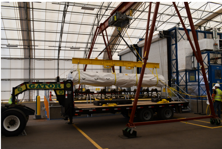
Waste Retrieval Operations crew prepare a CMP filled with cemented TRU waste for size-reduction using a 10-ton electric hoist mounted on a gantry and pipe rollers in Dome 375 at Technical Area 54.
