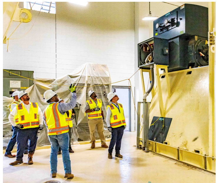
EM Principal Deputy Assistant Secretary Jeffrey Avery (left) is shown the 1,000-horsepower fan motor on a tour of the New Filter Building.
