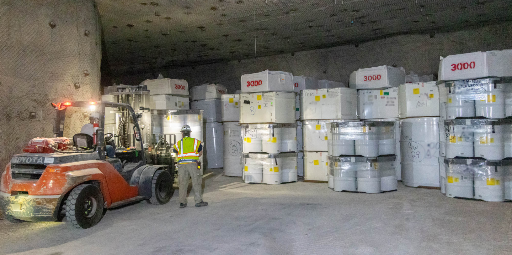
Workers emplace TRU waste containers in Room 2 of Panel 8 in the WIPP underground.
