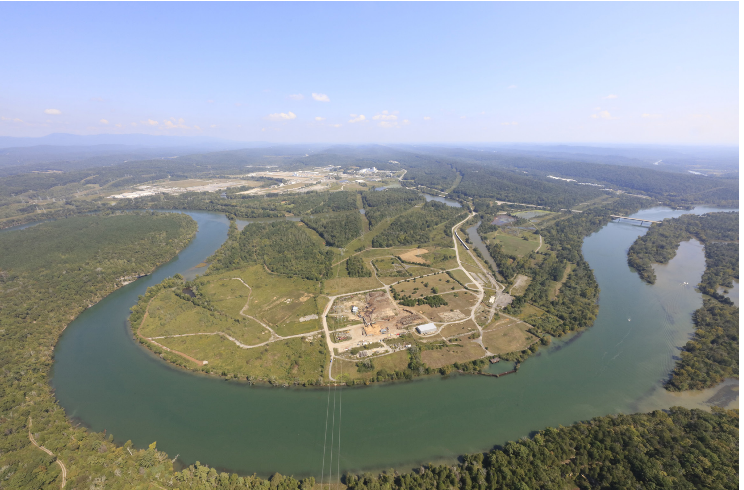
Aerial photo of the ETTP, where OREM has recently transferred 376 additional acres for economic development.
