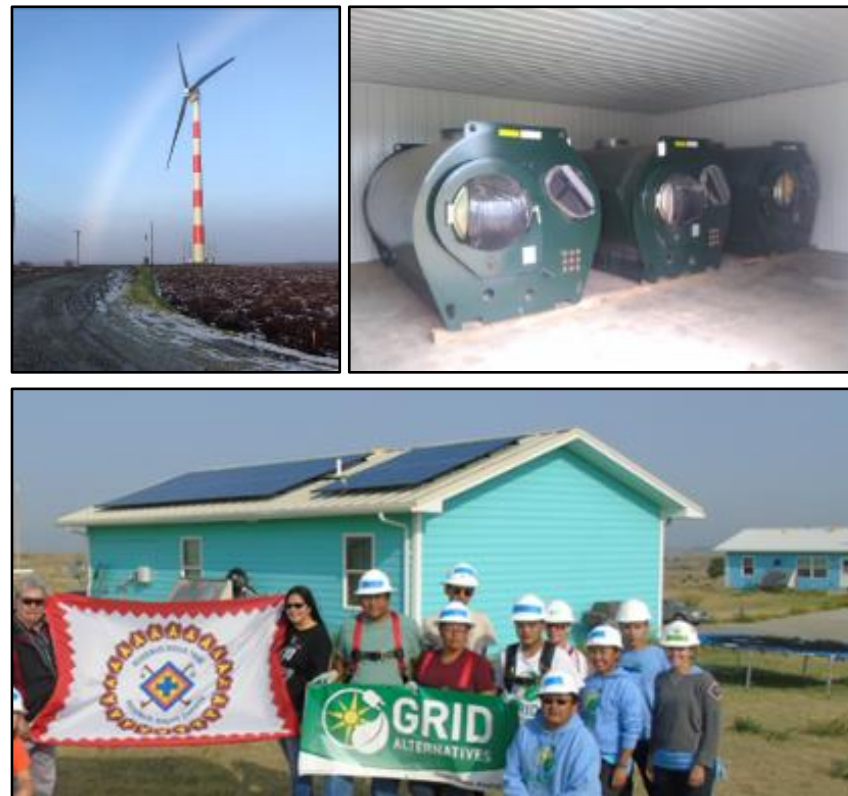
Clockwise from top right: Huslia Tribe Council (AK) installed a community-scale biomass project to heat their community's buildings (2018); Rosebud Sioux (SD) solar system on low-income home (2016); Alaska Village Electric Cooperative, Inc. (AVEC) and Bethel Native Corporation's (BNC) installed a 900-kW turbine to power the communities of Bethel and Oscarville, AK.
