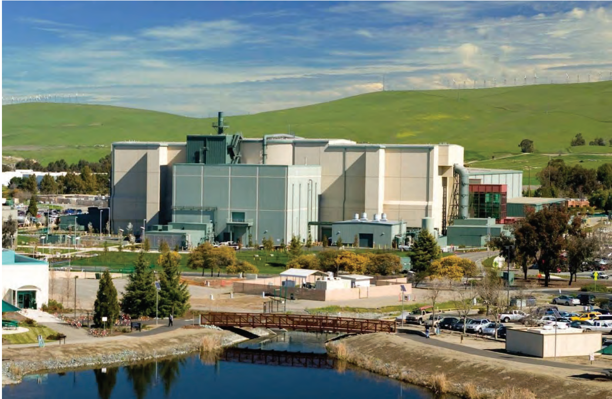
Figure 4-22. View of the NIF Looking Northeast
