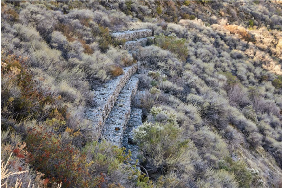
Figure 4-27. Gabion Retaining Walls
