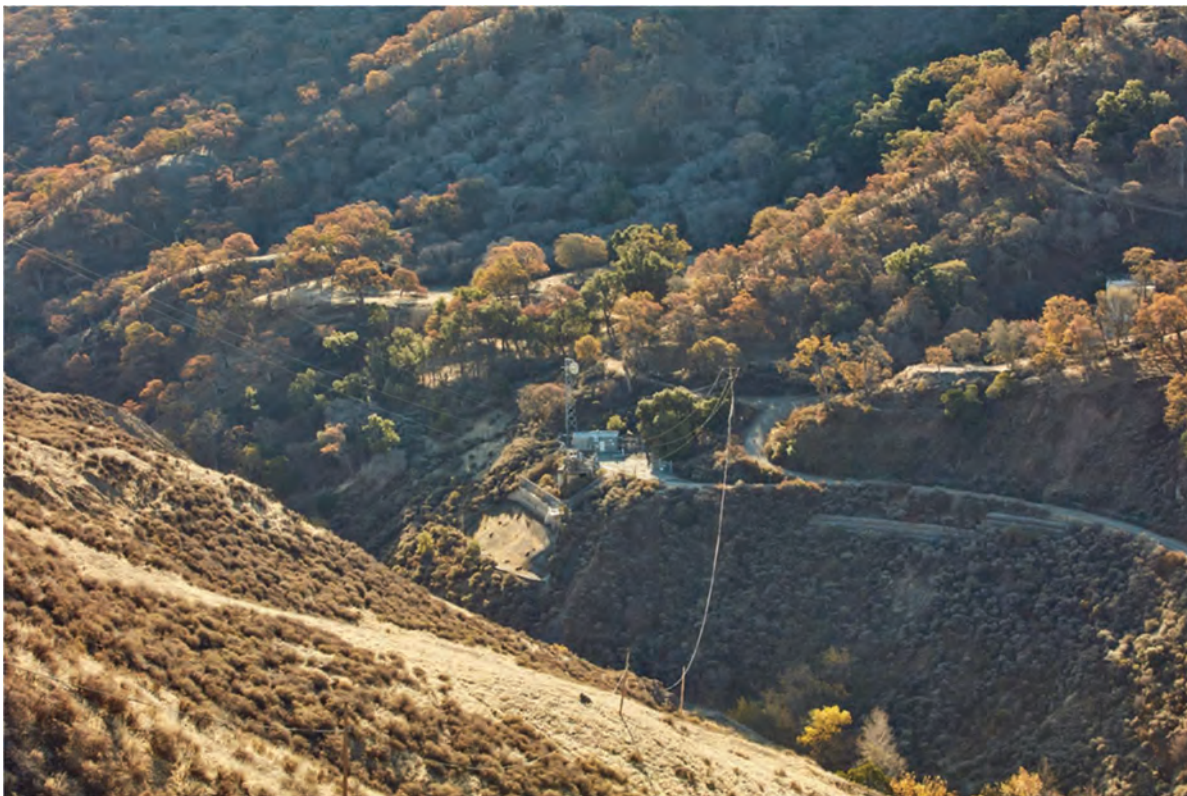
Figure 4-26. Arroyo Mocho Pump Station
