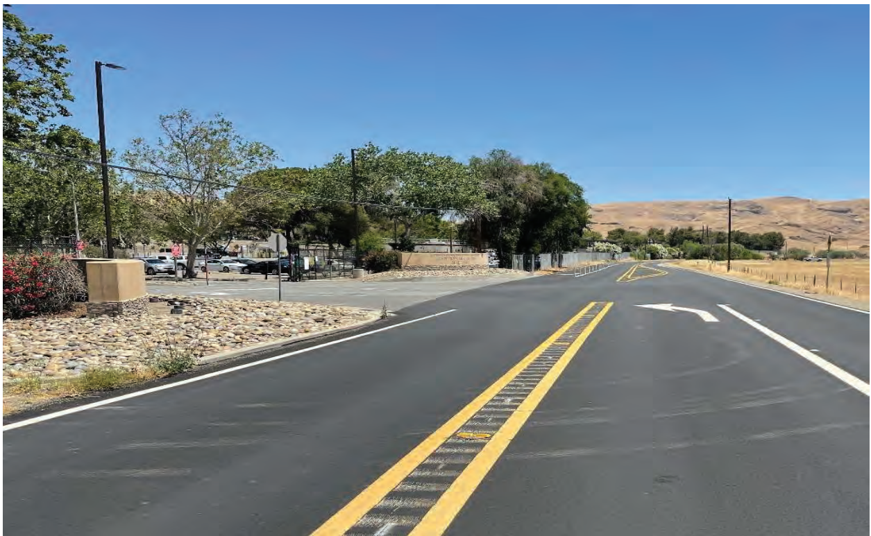
Figure 4-25. View of Site 300 GSA Entrance from Corral Hollow Road, Looking East
