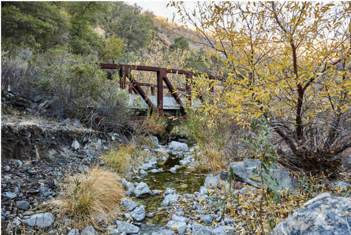
Figure 4-28. Steel Bridge to Arroyo Mocho Pump Station
