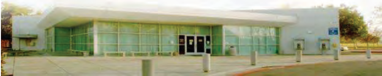
Figure 2-10. West Gate Badge Office
