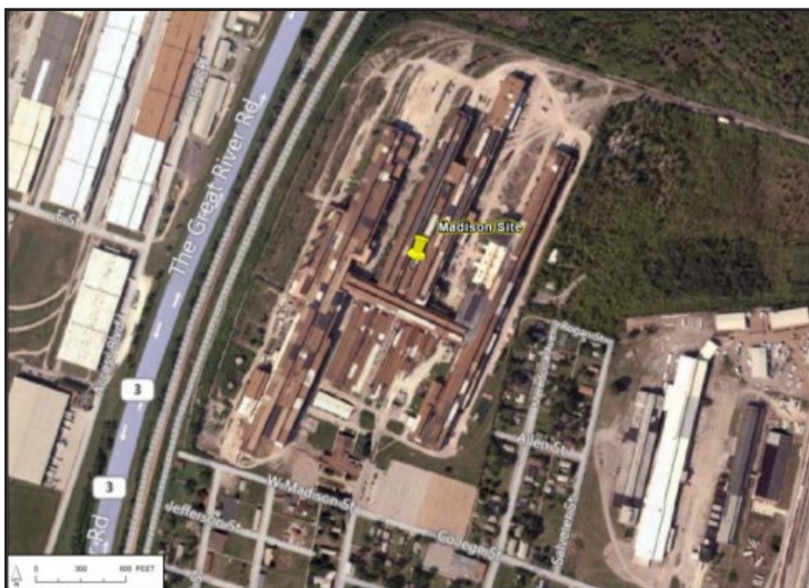
Aerial view of the Madison site.
