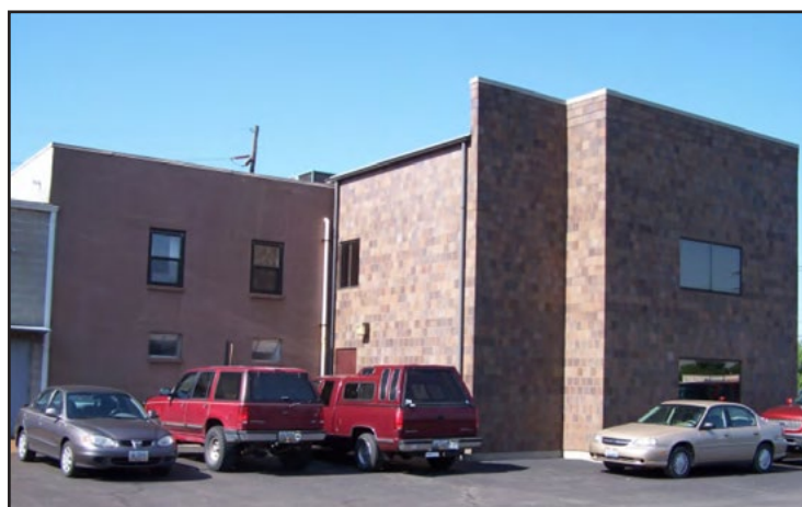
New building addition at the Fairfield, Ohio, Site (May 2006).
