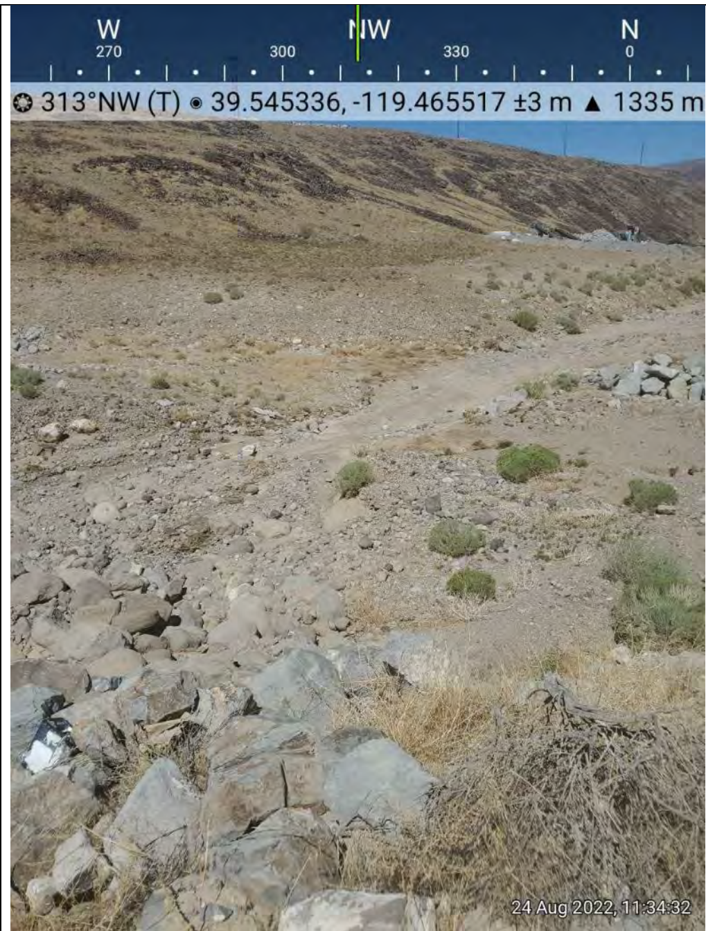
Photo 3. Looking downstream at AR 1 after passing through culverts.
