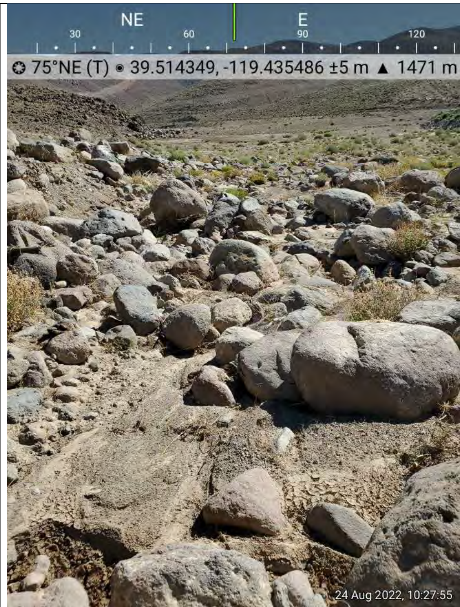
Photo 4. AR 1 looking downstream through detention basin entering the first of a series of 4 rock check dams.
