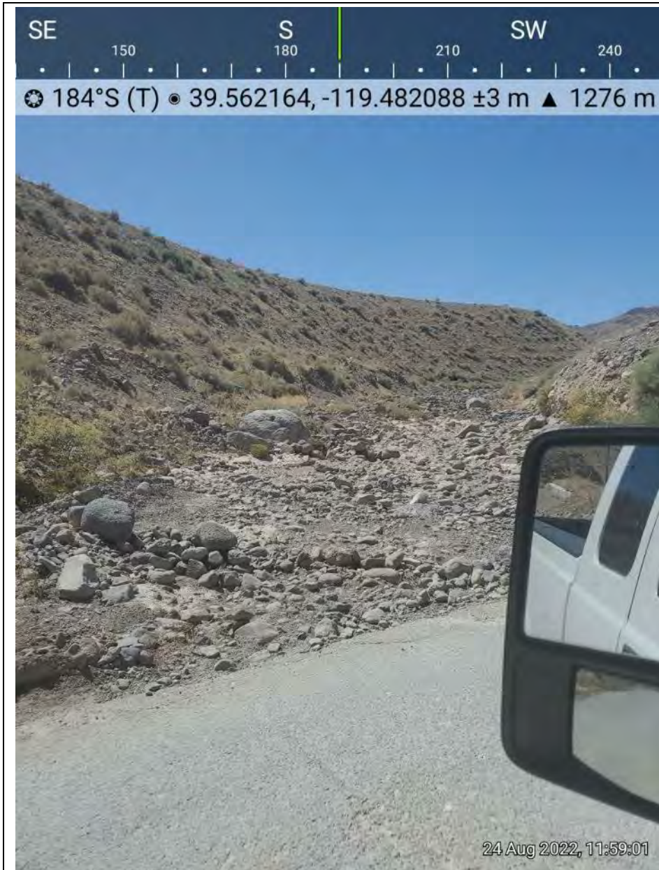
Photo 1. Looking upstream at AR 1 from Clark Station Road, a publicly accessible roadway.
