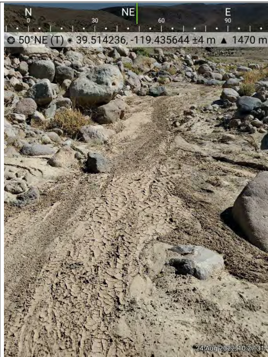
Photo 4. AR 1 looking downstream through detention basin approaching first of a series of 4 rock check dams.
