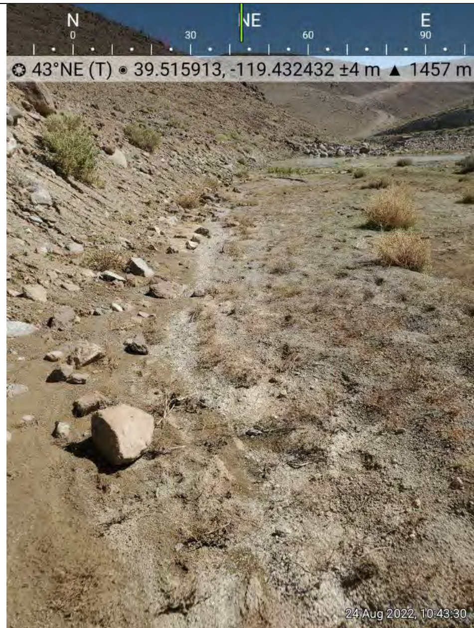
Photo 18. AR 1 through retention basin towards rock check dam #4.
