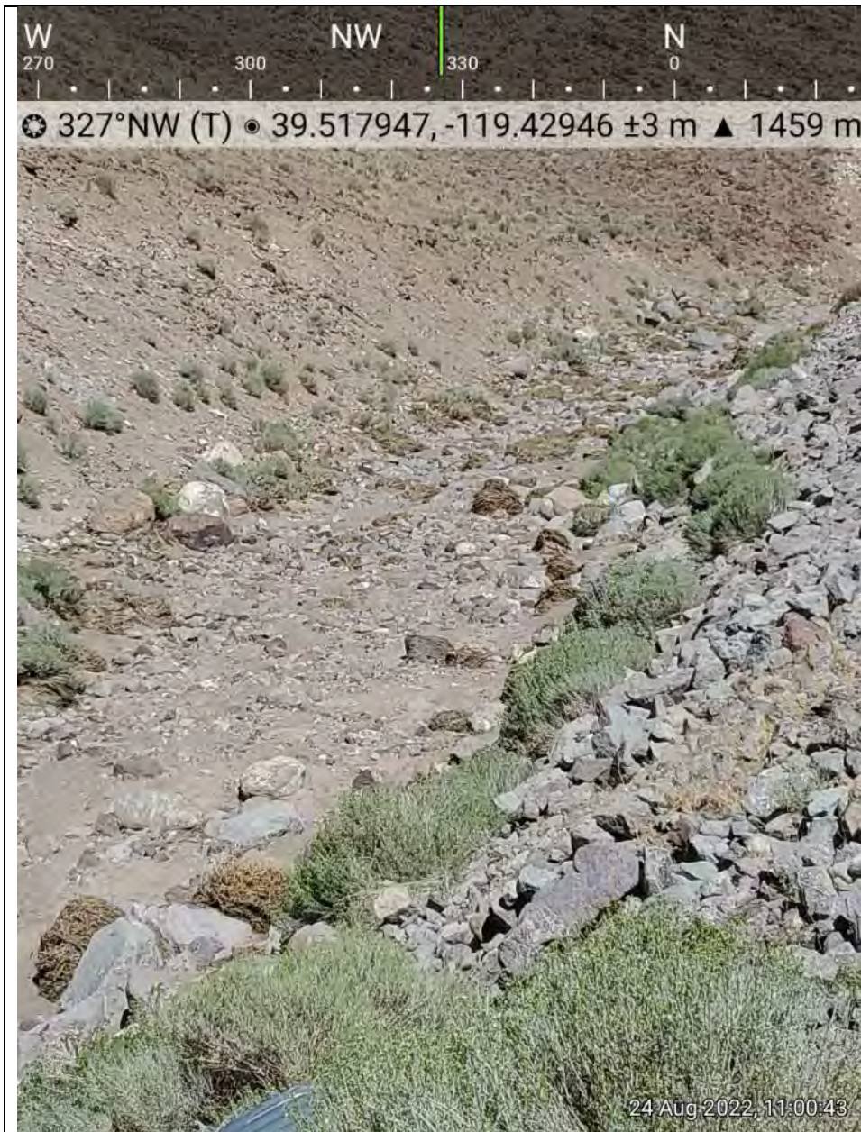
Photo 3. Looking at AR 1, downstream of confluence with second set of culverts.
