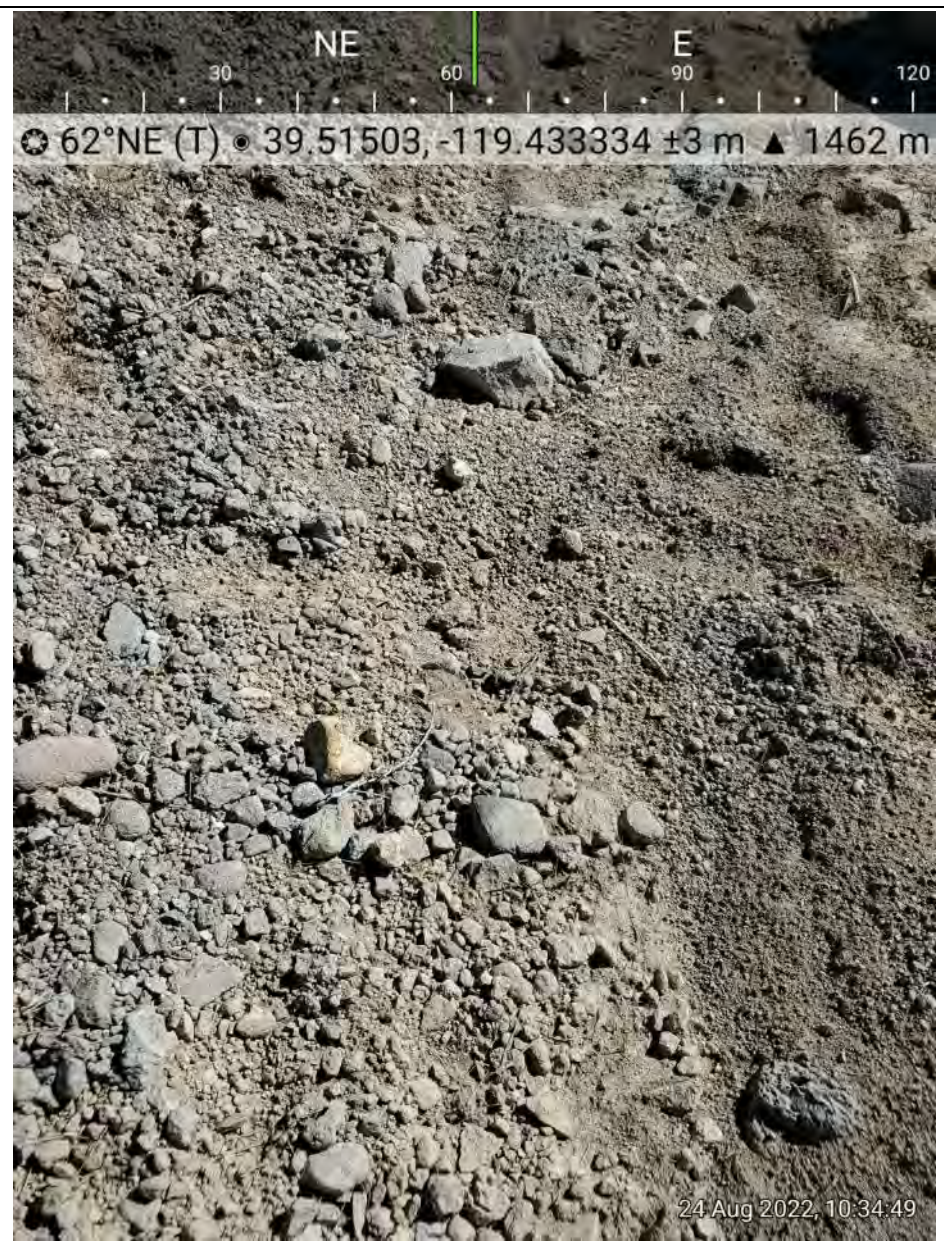
Photo 10. AR 1 out of rock check dam #2 and into next retention basin.
