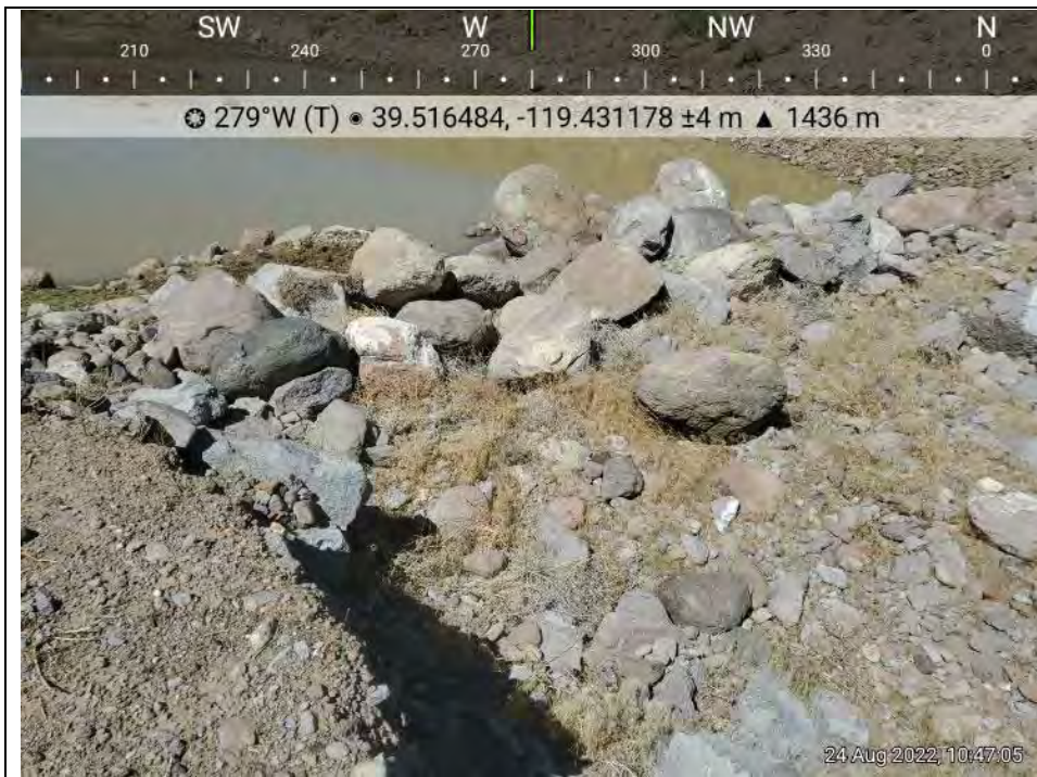
Photo 21. Looking upstream at AR 1 from top of rock check dam #4.
