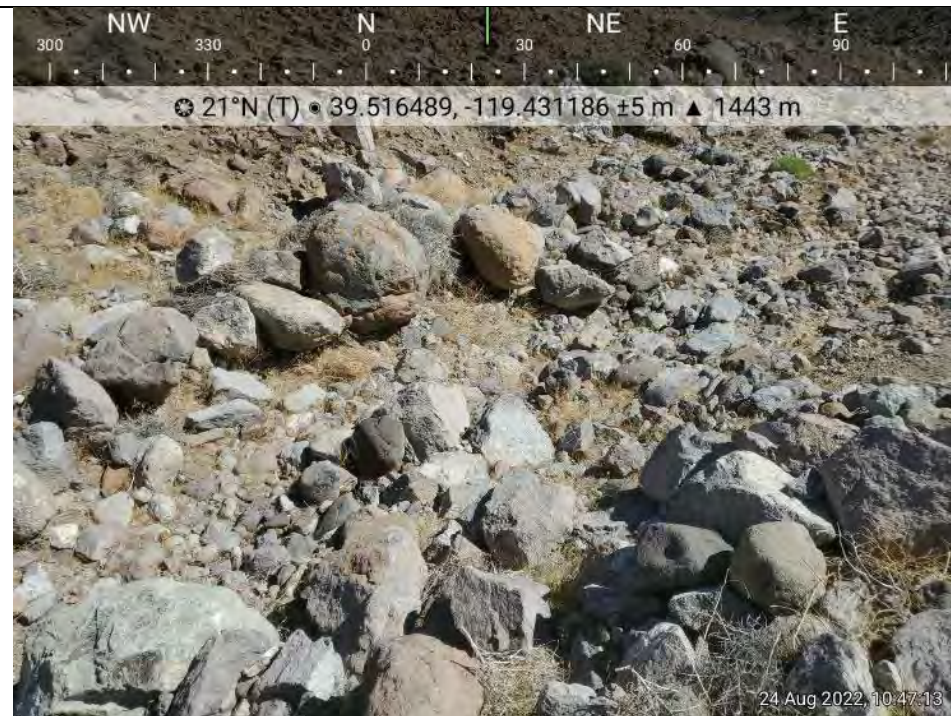
Photo 22. Looking downstream at back of rock check dam #4.
