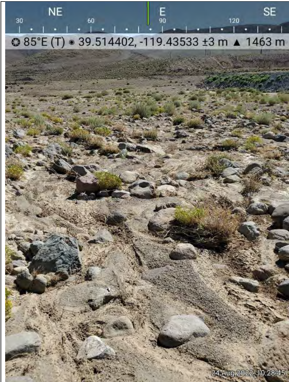
Photo 1. AR 1 out of rock check dam #1 and into next retention basin.
