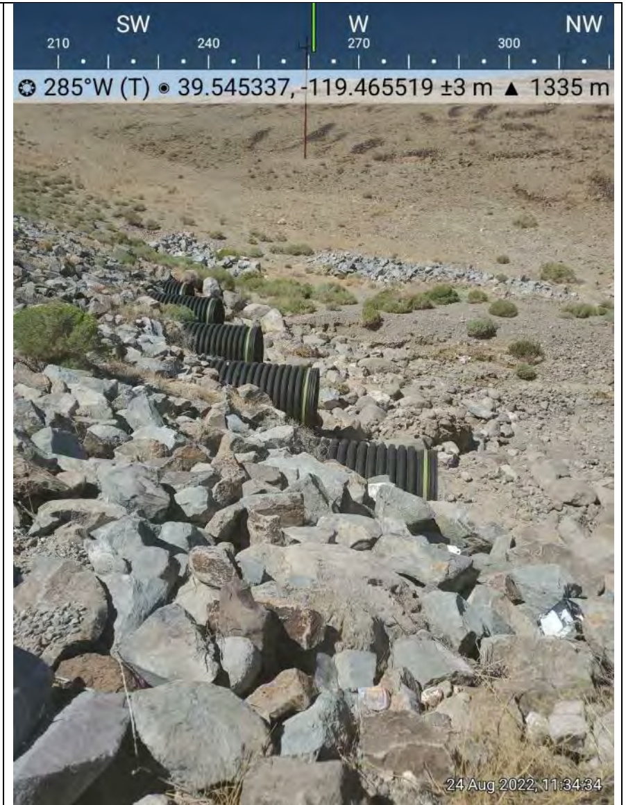
Photo 2. Looking at downstream outlet of culverts passing under public roadway.
