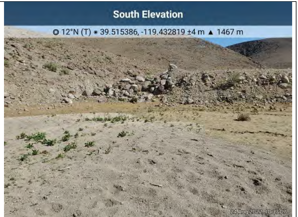
Photo 12. AR 1 through retention basin and towards rock check dam #3.
