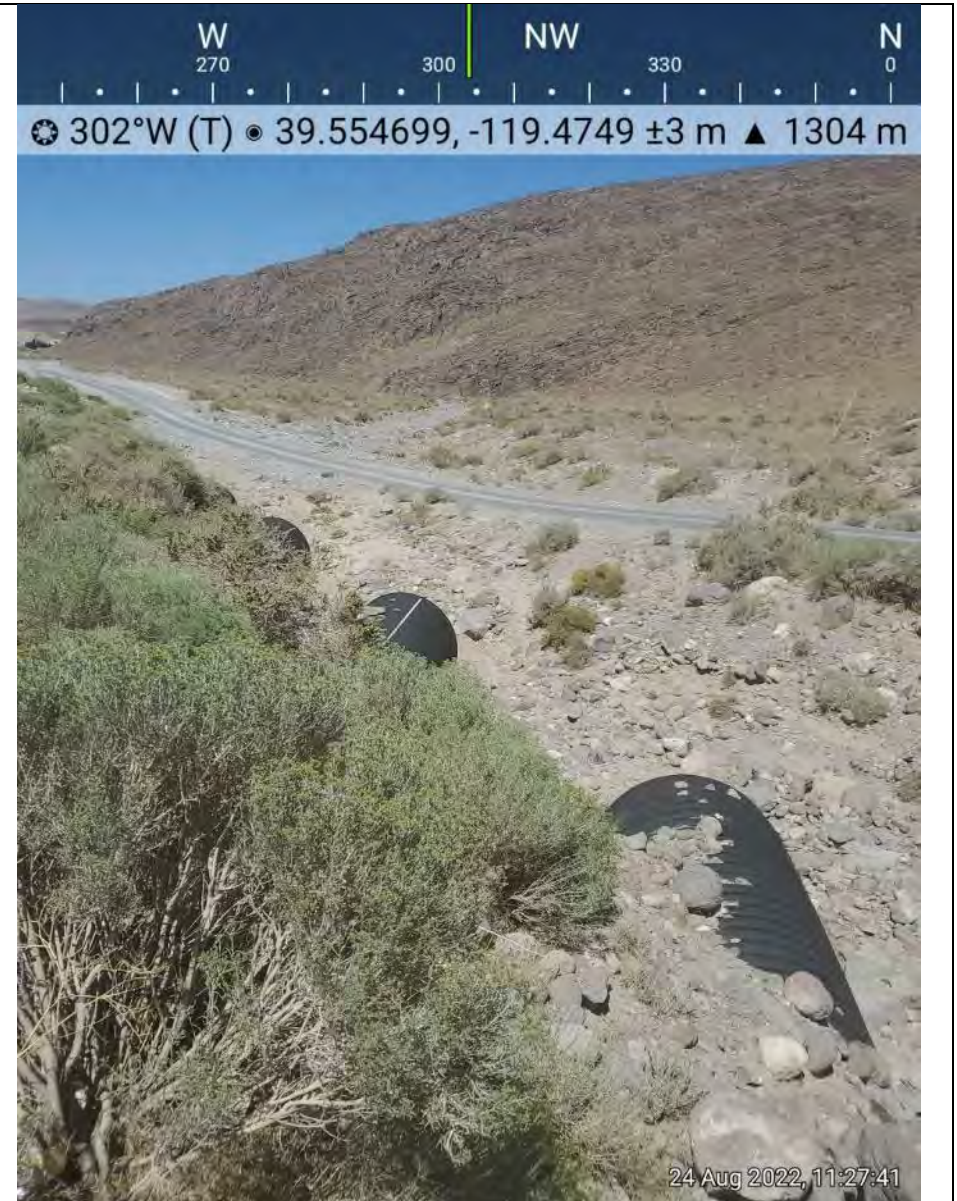
Photo 2. Looking downstream at AR 1 after culverts pass under Electric Avenue. Roadway constructed through AR 1 is privately owned and inaccessible. No evidence of flow across that roadway.
