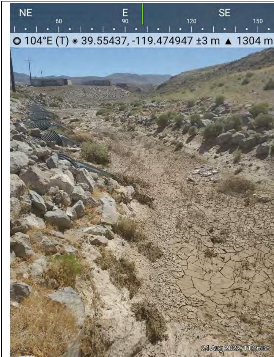
Photo 1. Looking upstream at AR 1 from public roadway. Evidence of impounded water that has evaporated, but there was no evidence of flow through the culverts to the other side of Electric Avenue.
