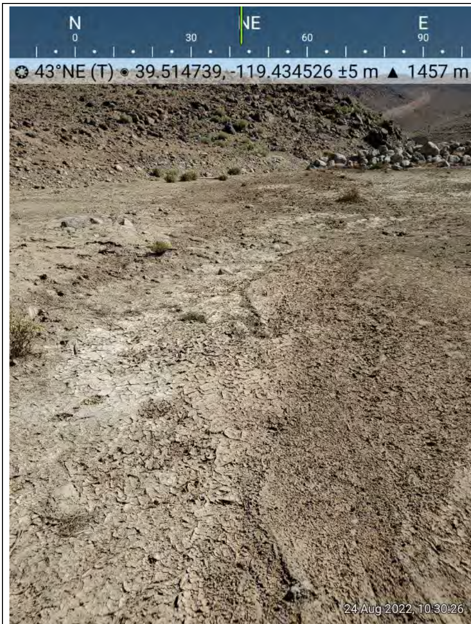
Photo 5. AR 1 through retention basin and towards rock check dam #2.
