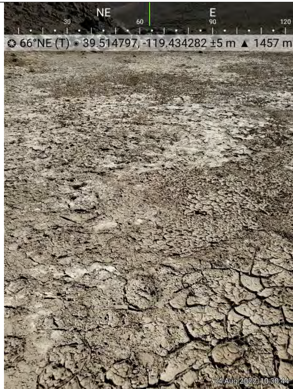
Photo 6. AR 1 through retention basin and towards rock check dam #2. Mud cracks indicative of recent evaporation following August precipitation.
