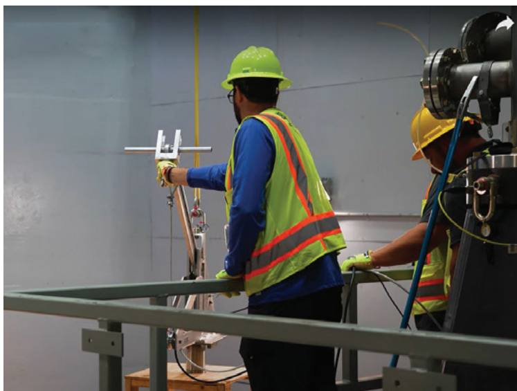
Testing the mechanical arm planned for use at Building 3517
