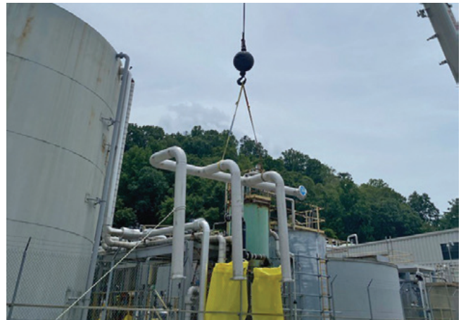
Pipe replacement at Building 3608
