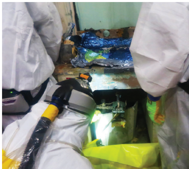
HEPA filter hood removal in Building 3030, Isotope Row
