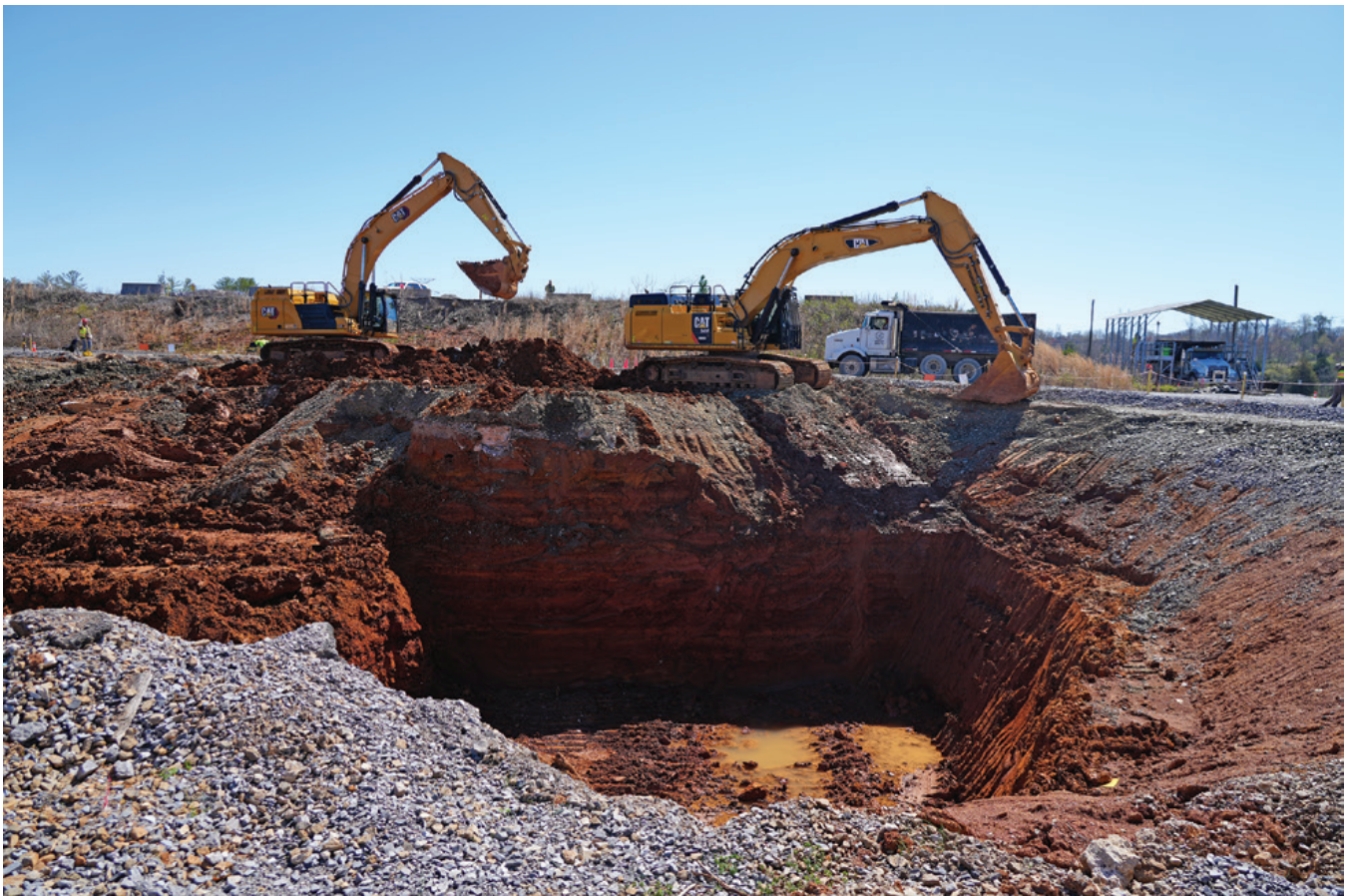
Excavation activities at EU-13
