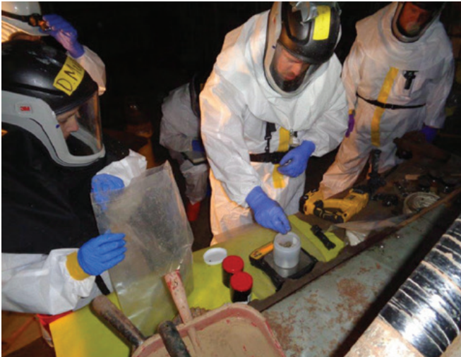
Workers perform sampling activities inside the Alpha-2 Building
