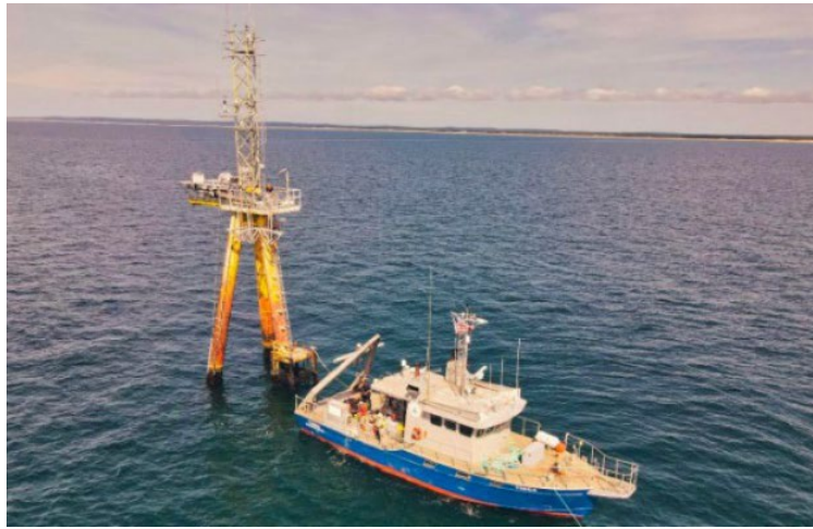
Figure 4. Existing ASIT Tower site where instrument installations will take place.
