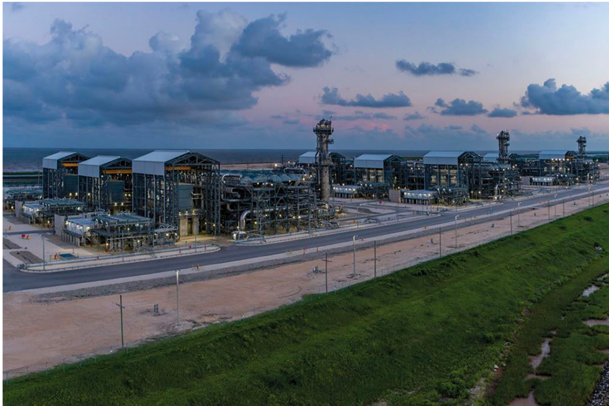
The Freeport liquefied natural gas facility in Texas. Freeport LNG via Business Wire
