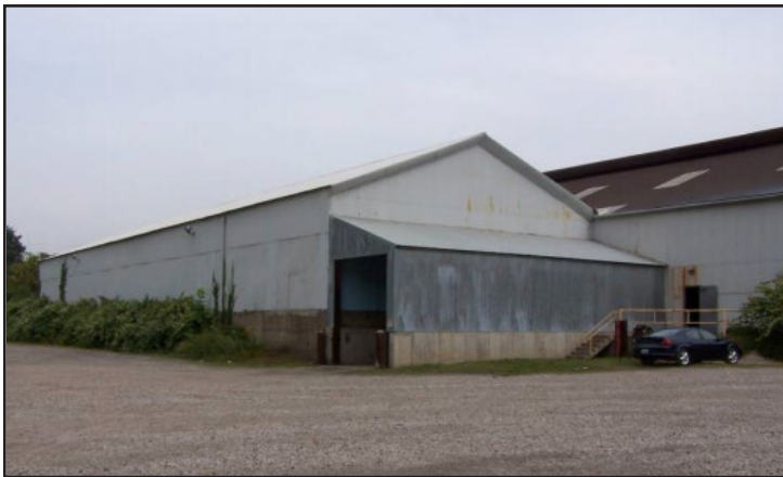
Front of remediated building at the Aliquippa site (September 2005).
