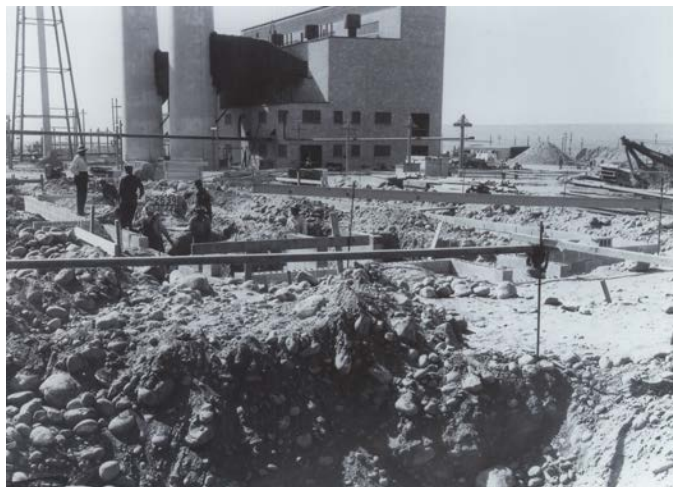
Historical photo: Hanford 184-B Power House under construction. Provided steam for heating and processing to the B Reactor and surrounding support facilities.
