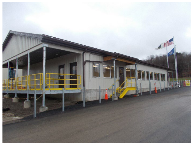
Guard House on November 28 , 2022
