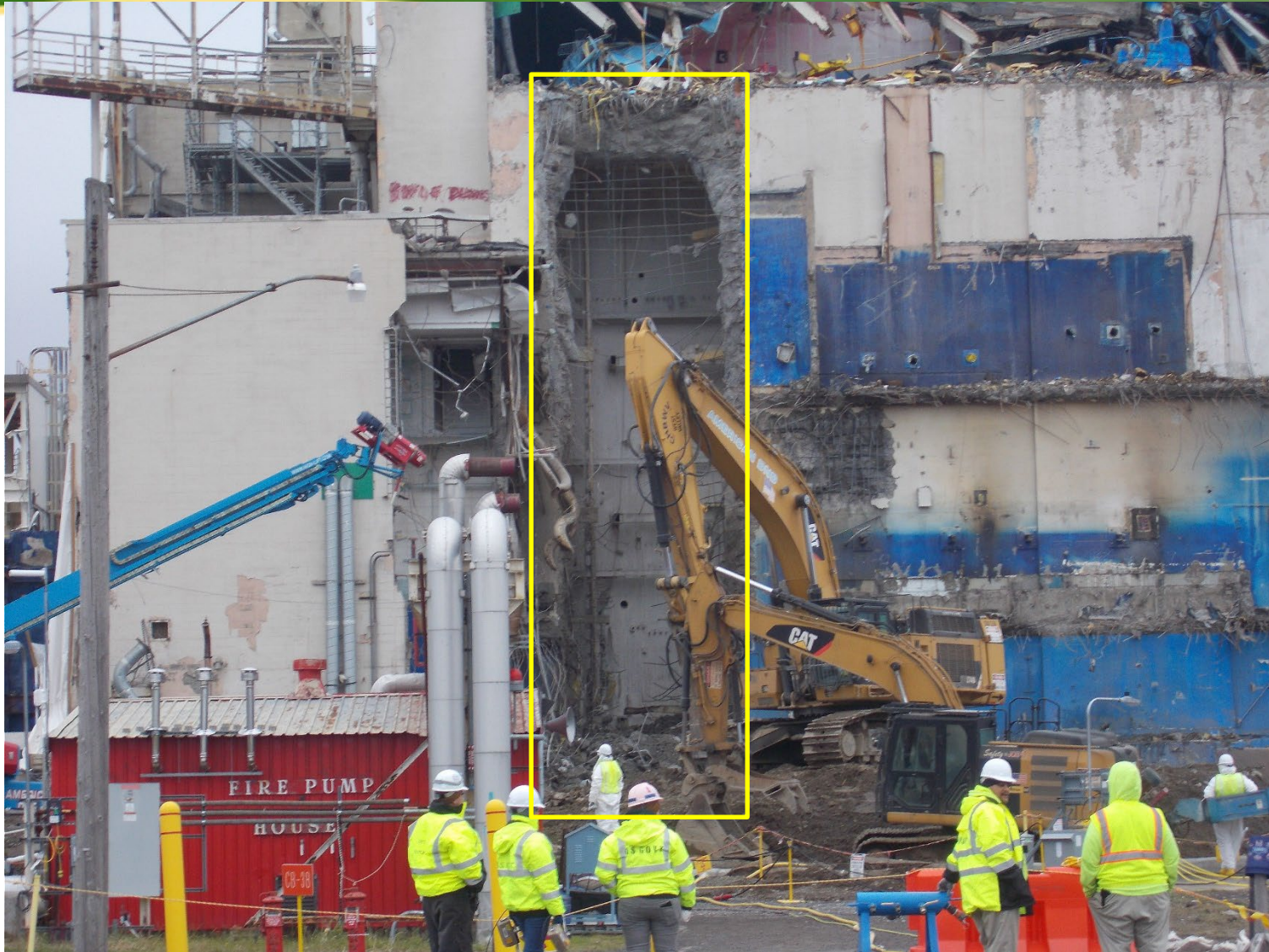
Deconstruction of Extraction Cell #1
