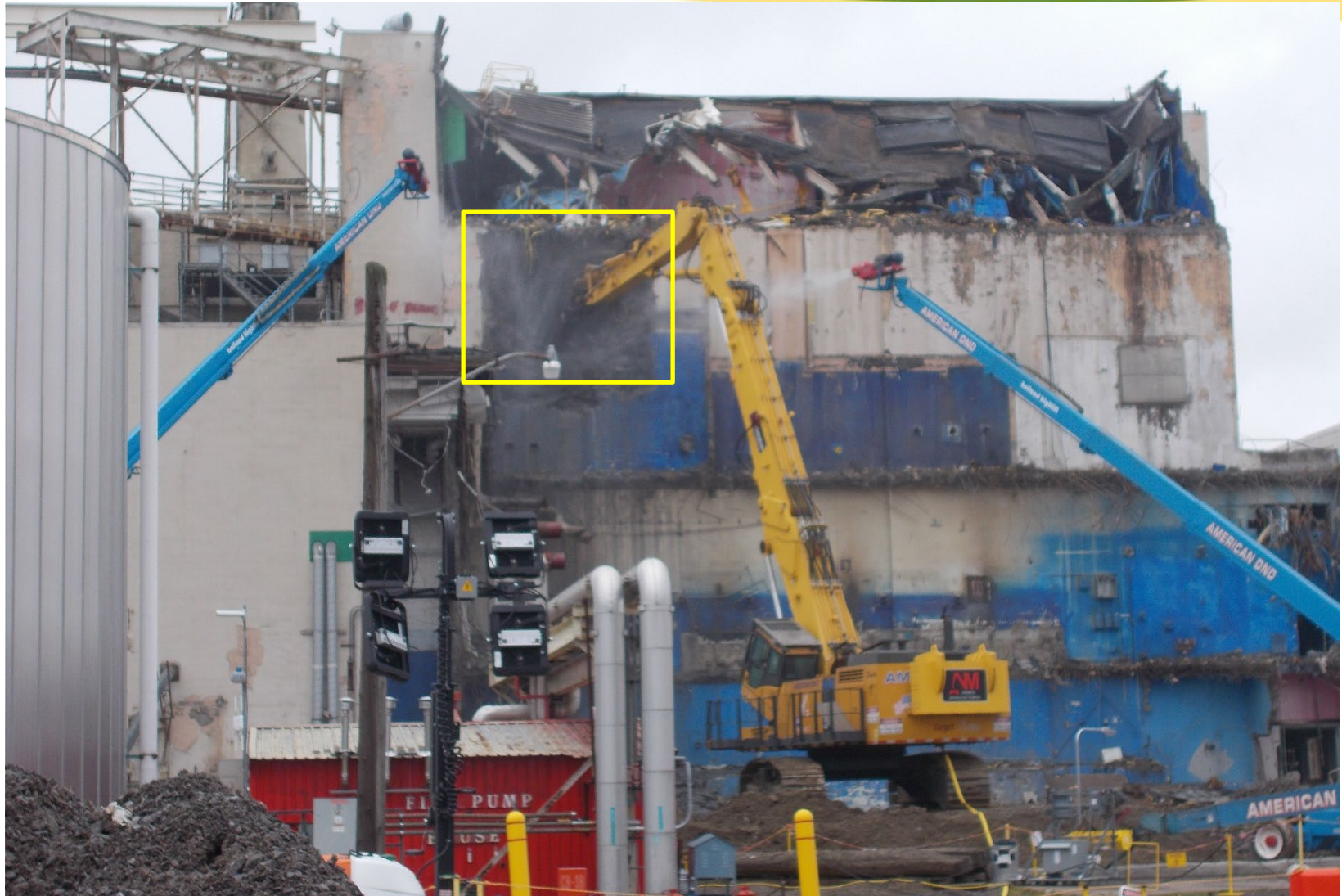
Deconstruction of Extraction Cell #1
