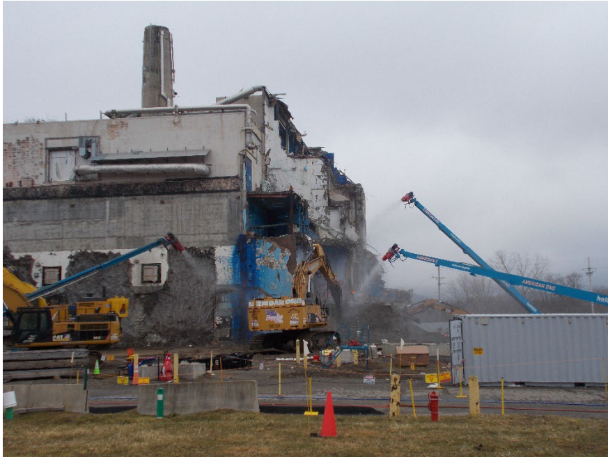
Deconstruction of Acid Recovery Cell – Off-Gas Operating Aisle
