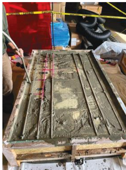
Figure II.3.3.3. Grout poured uniformly across the encasement of the 200 kW DWPT transmitter.
