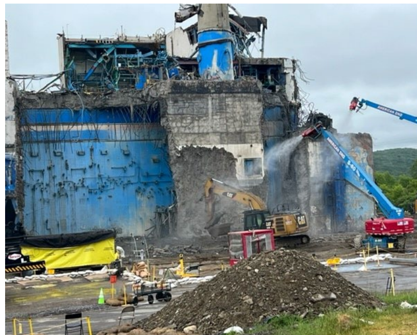
Deconstruction of Chemical Process Cell, managing the debris pile (June 12)
