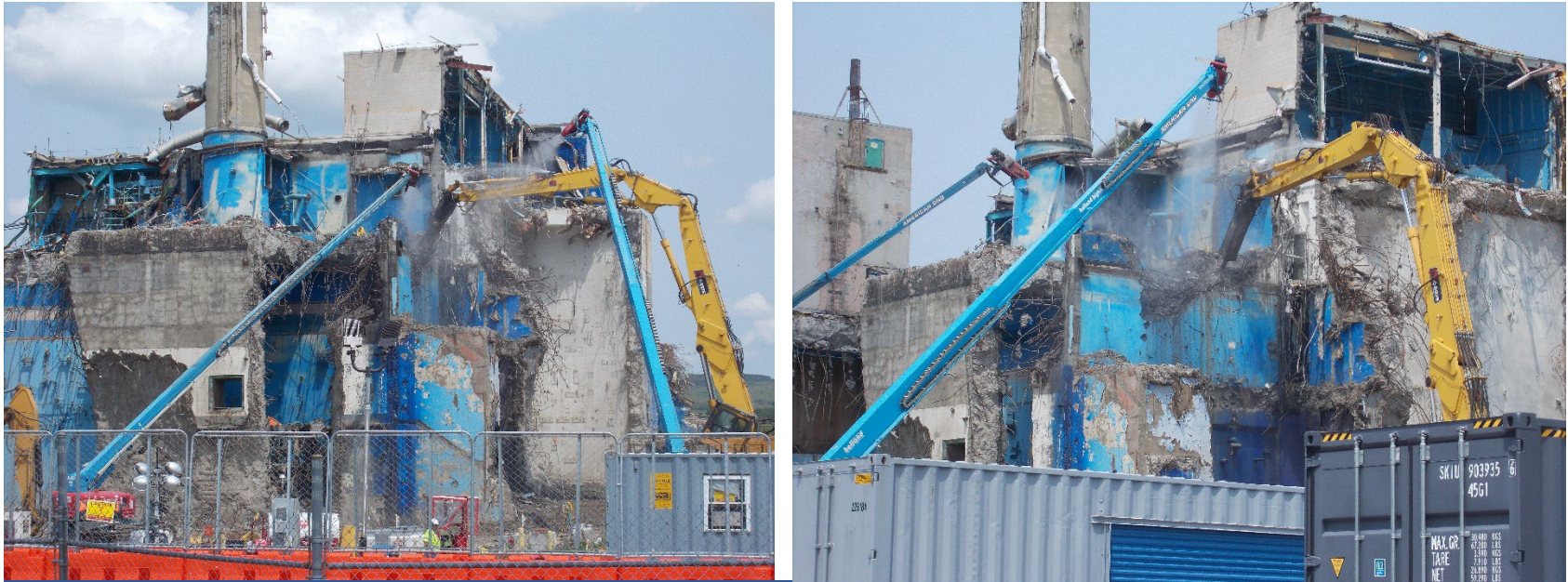
Deconstruction of Chemical Process Cell south wall (May 22)
