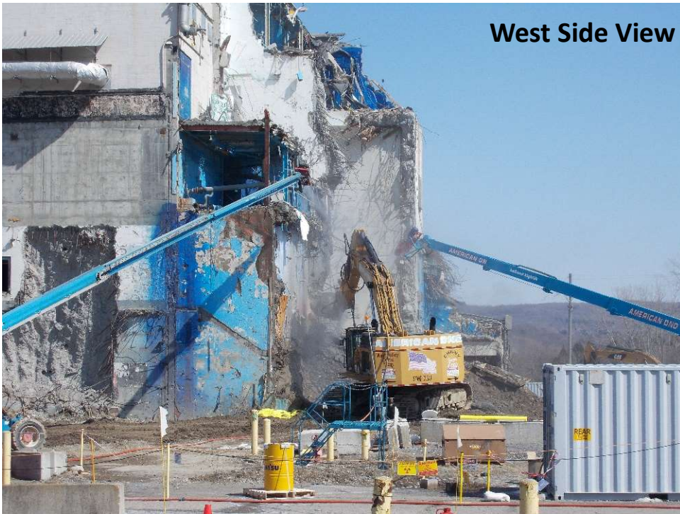
Deconstruction of Extraction Cell #1's 5-foot thick reinforced concrete west wall
