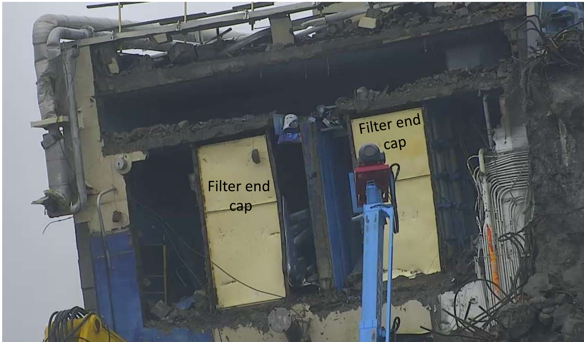
Deconstruction of Ventilation Exhaust Cell
