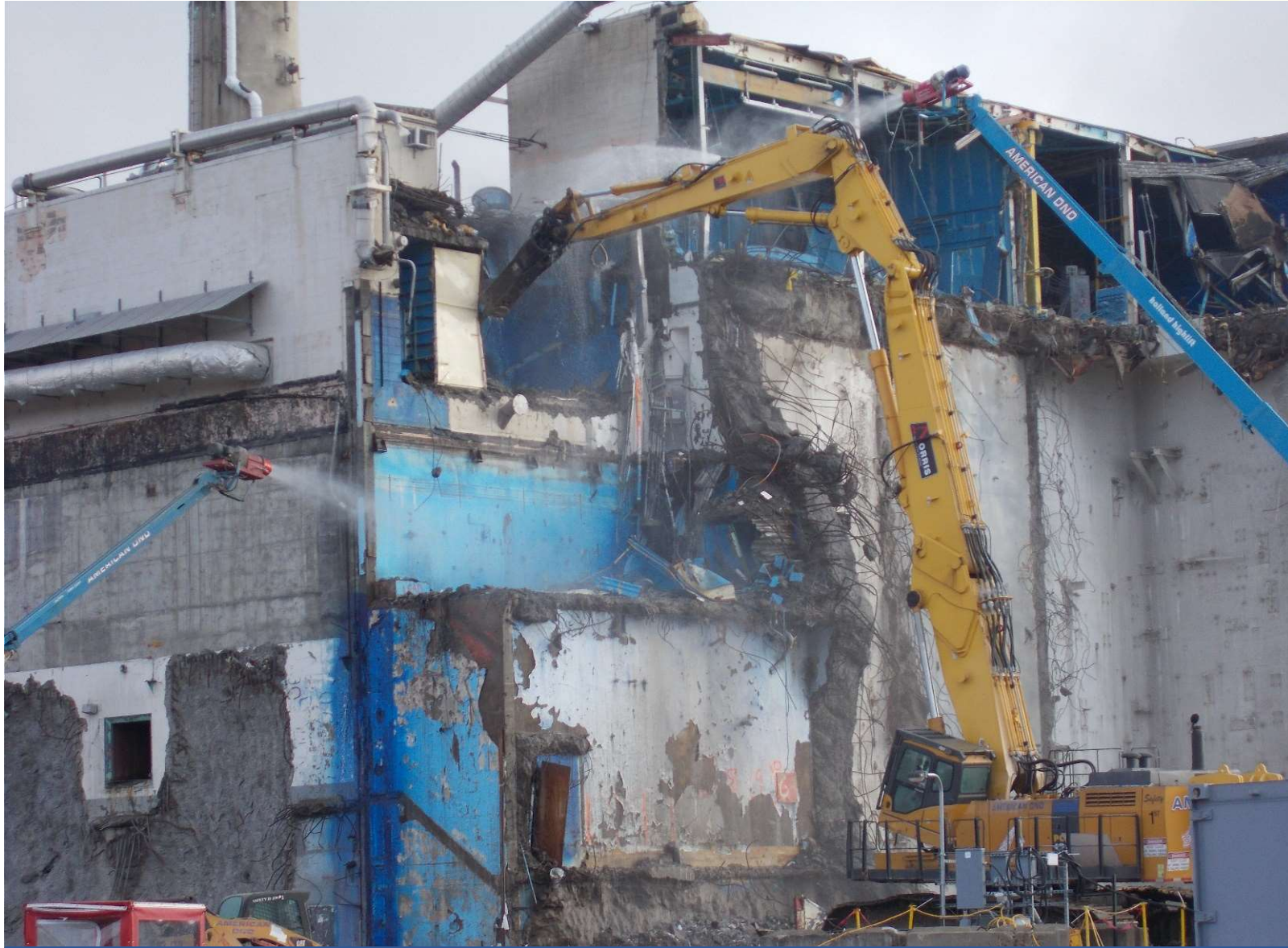
Deconstruction of Ventilation Exhaust Cell
