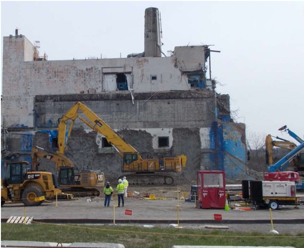
Staging equipment on the west side to dismantle Hot Acid Cell and Process Chemical Room
