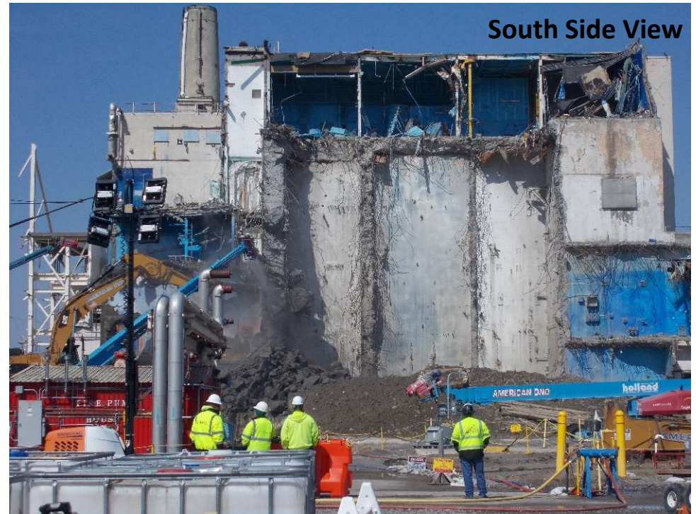
Deconstruction of Extraction Cell #1's 5-foot thick reinforced concrete west wall
