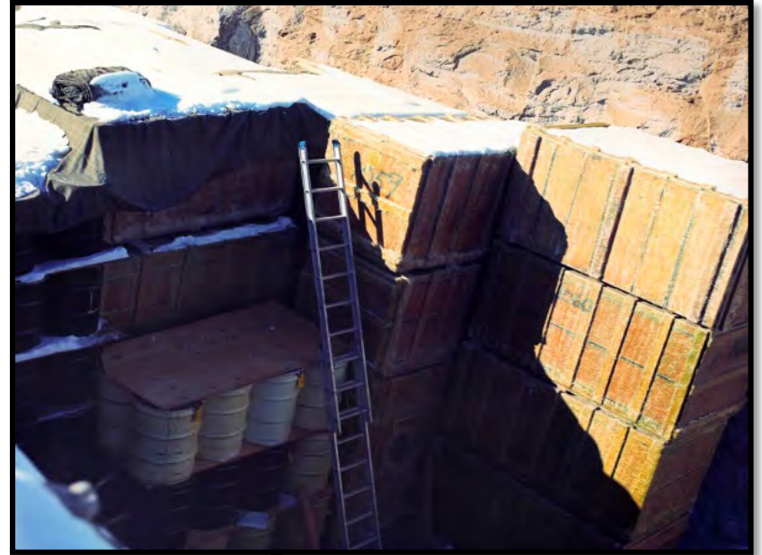
Fiberglass-reinforced Plywood Boxes in Pit 9
