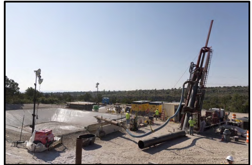
Drilling Operations for Groundwater Monitoring Well R-71
