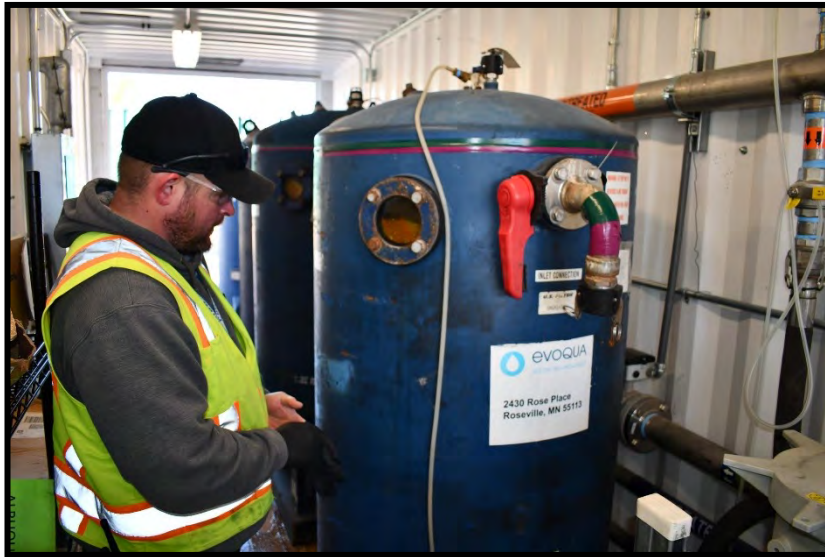
Ion Exchange Unit Where Groundwater Contaminated with Hexavalent Chromium is Treated
