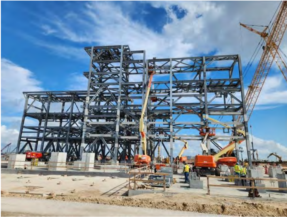
Photo 3: Area 311A01 Structural Steel (Train 1)
