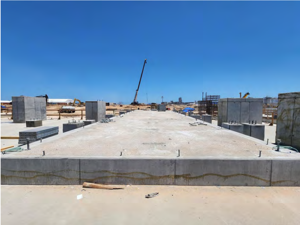
Photo 1: Area 311A02 Compressor Foundation (Train 1)
