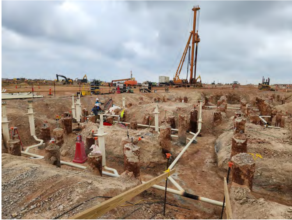
Underground Amine Pipe Installation in Train 1
