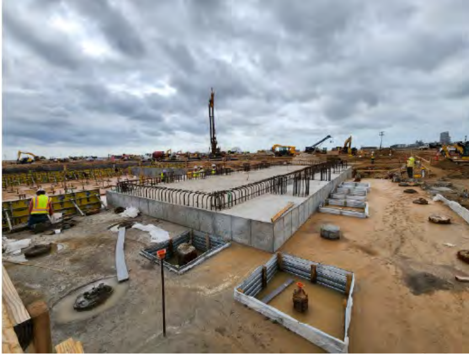
Photo 5: Train 1 Compressor Foundation progress
