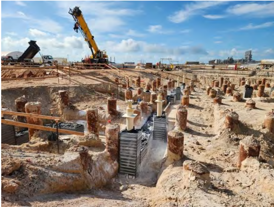
Photo 1: Area 311L01 Amine Pipe Installation - Gilsulate 500XR design (Train 1)
