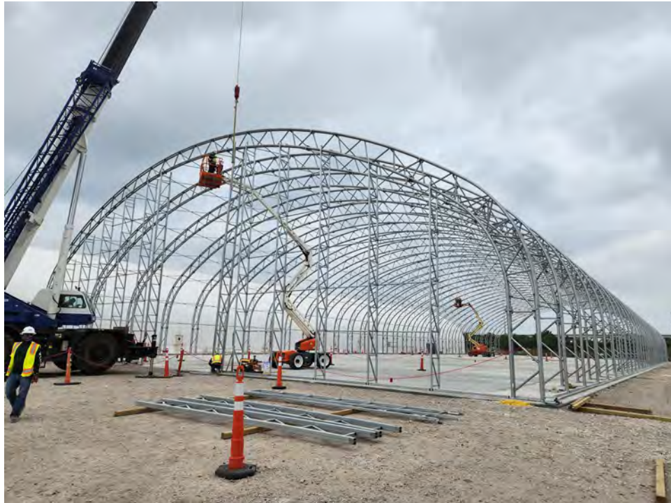
Procurement Warehouse #2 Steel Frame Erection
