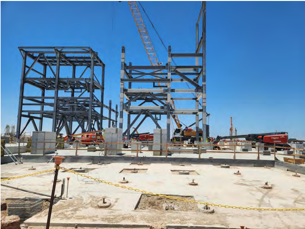
Photo 2: Area 311A01 Structural Steel (Train 1)
