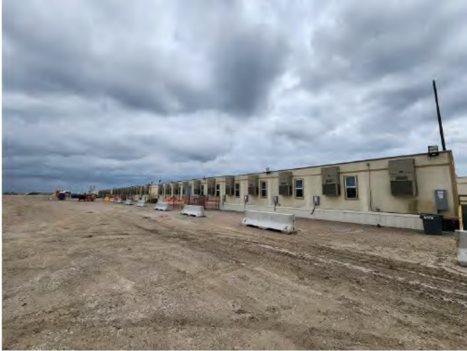
Photo 1: New Construction Management Trailer (CMT) Complex Nearing Completion
