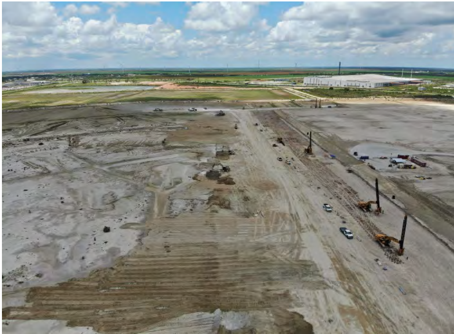
Photo 6: Soil Stabilization and Wick Drains in Zone 2b
