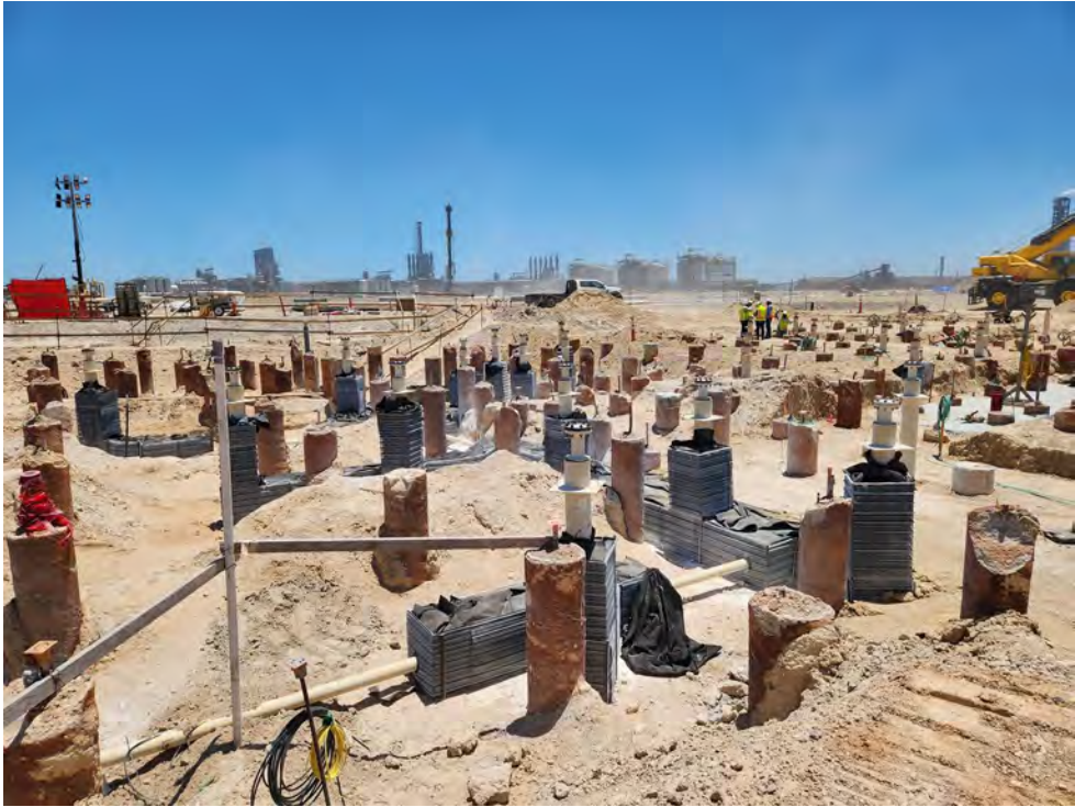
Photo 4: Underground Amine Pipe Installation (Train 1)
