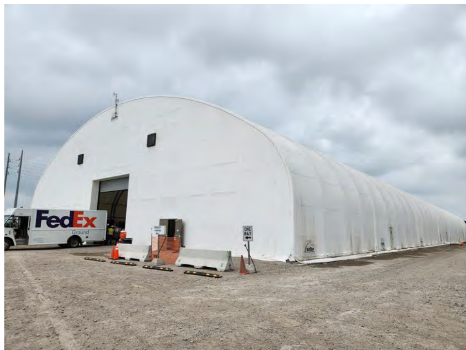
Procurement Warehouse #1 ready for Receiving
