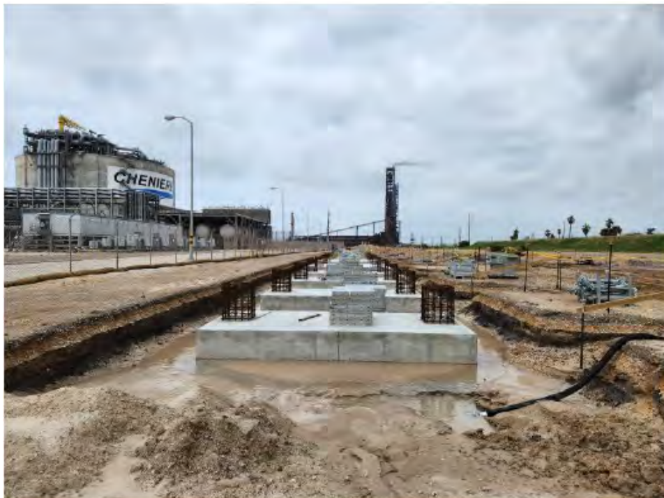
Photo 4: Concrete Foundations progress in OSBL South
