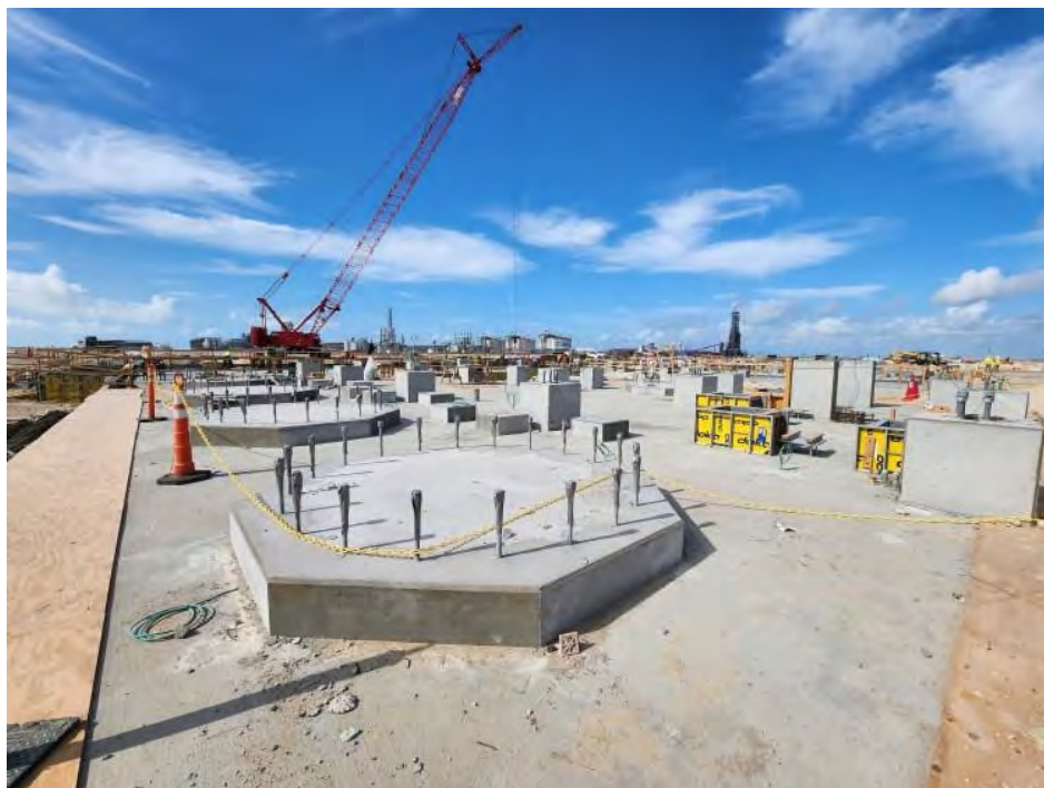
Photo 2: Area 311F01 Foundations (Train 1)
