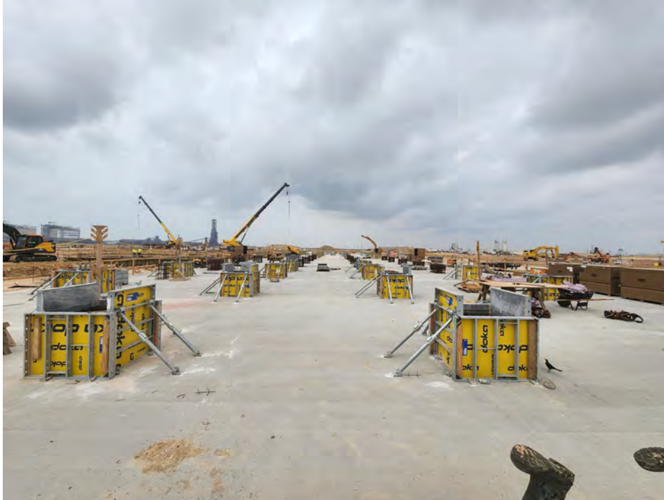
Train 1 Cryogenic Rack Area Foundations Complete and Pedestals in Progress
