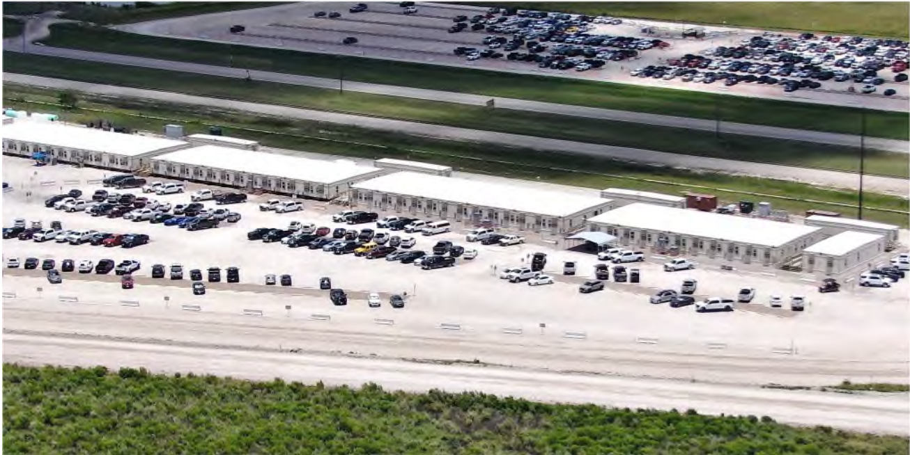
Photo 1: New CMT Complex occupied
