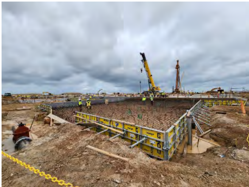
Photo 6: Train 1 Cold Box Foundations progress
