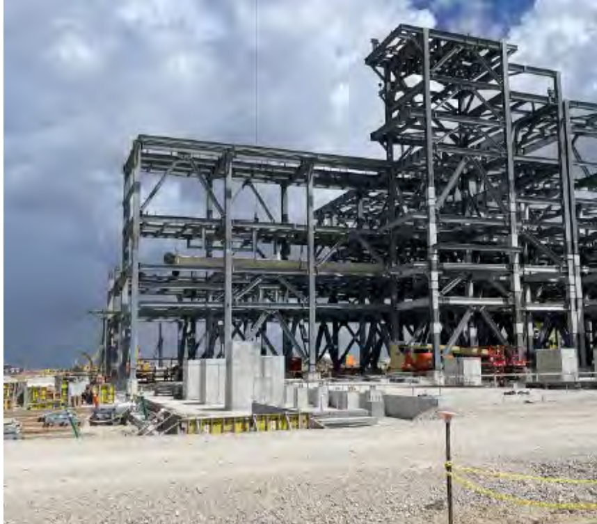
Photo 1: Area 311A01 Cryo Piperack — first spools in rack (Train 1)
