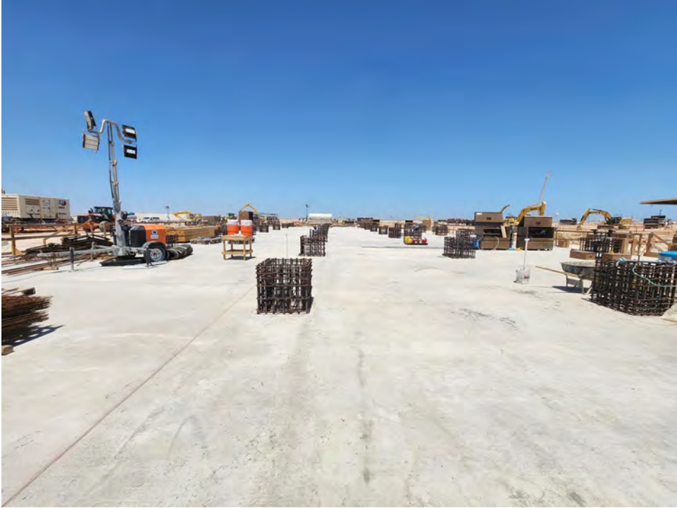
Photo 5: Area 322B01 Foundation progress (Train 2)
