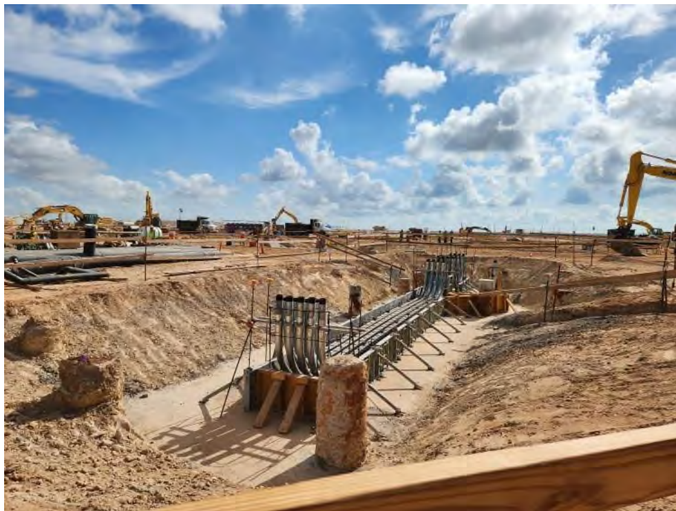
Photo 4: Duct bank installation (Train 2)
