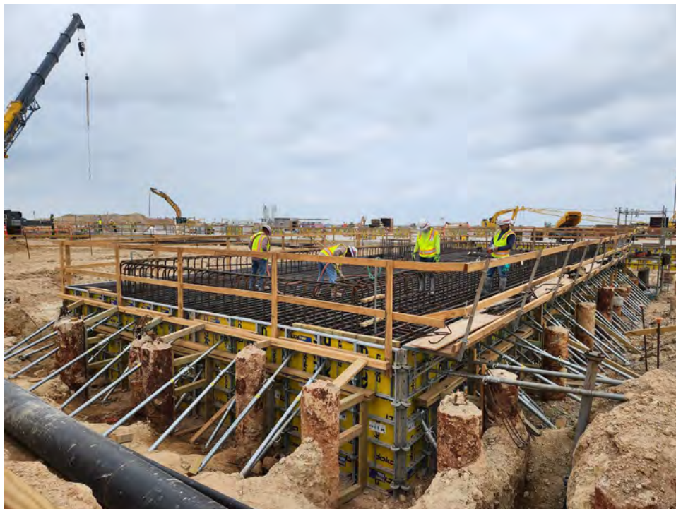
311B02 Compressor Foundation Rebar & Formwork
