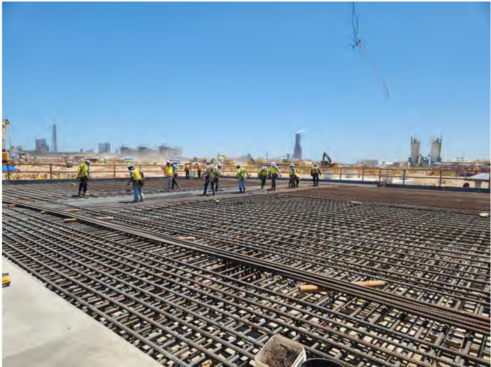
Photo 6: Area 322A01 Foundation Rebar (Train 2)
