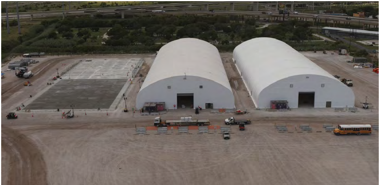
Photo 2: Procurement Warehouses #1 and #2 and foundation for Warehouse #3
