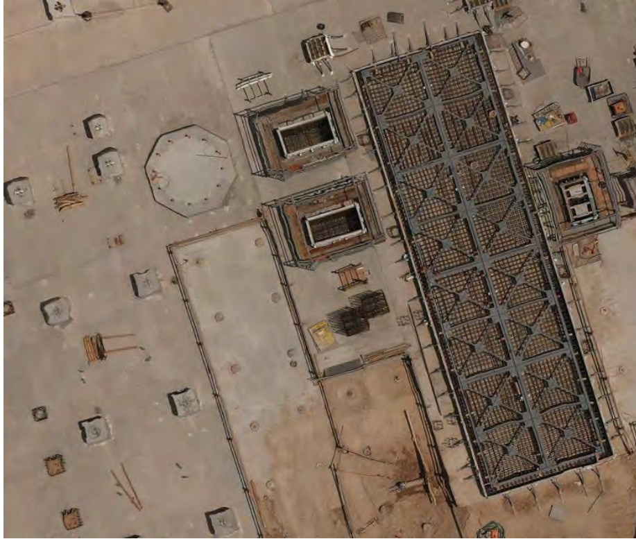
Photo 5: Train 1 Compressor Foundation progress (311B02)
