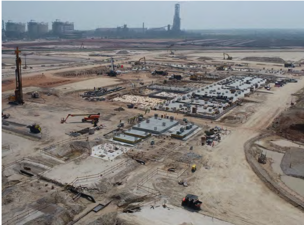
Photo 4: Concrete Foundations progress in Train 1
