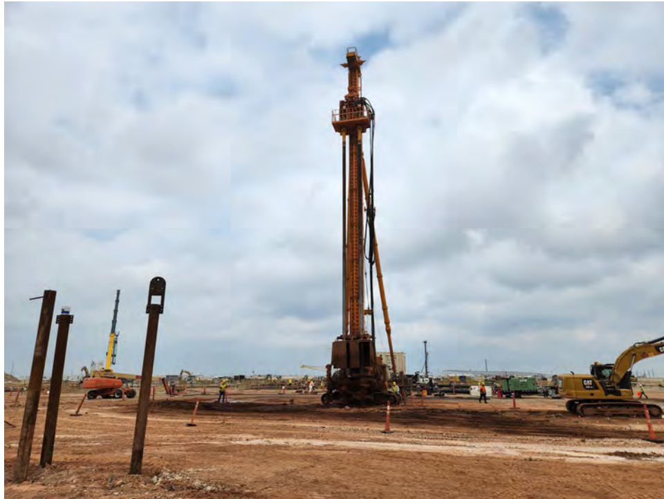
DMM rig at Train 1 (Amine storage/ISBL containment sump)
