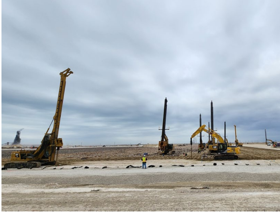
Wick drain installations progress in Train 7
