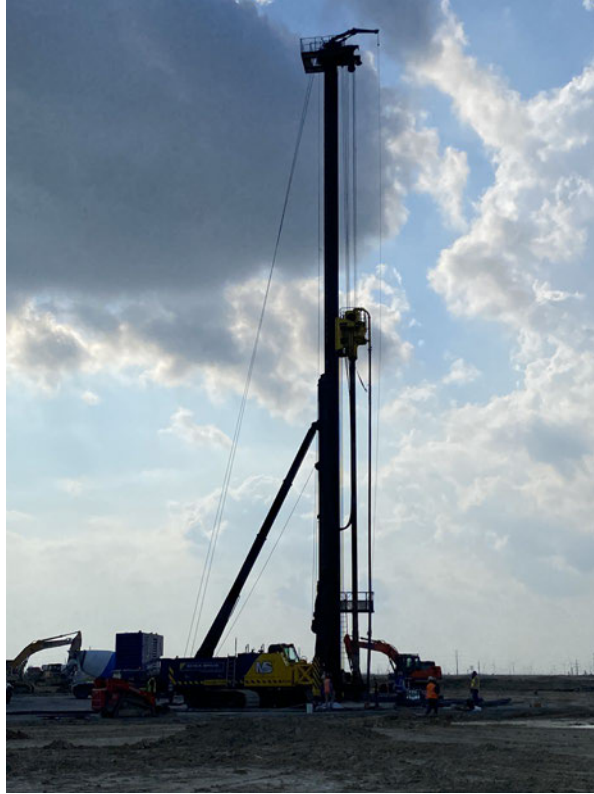
First pile installation on September 12, 2022
