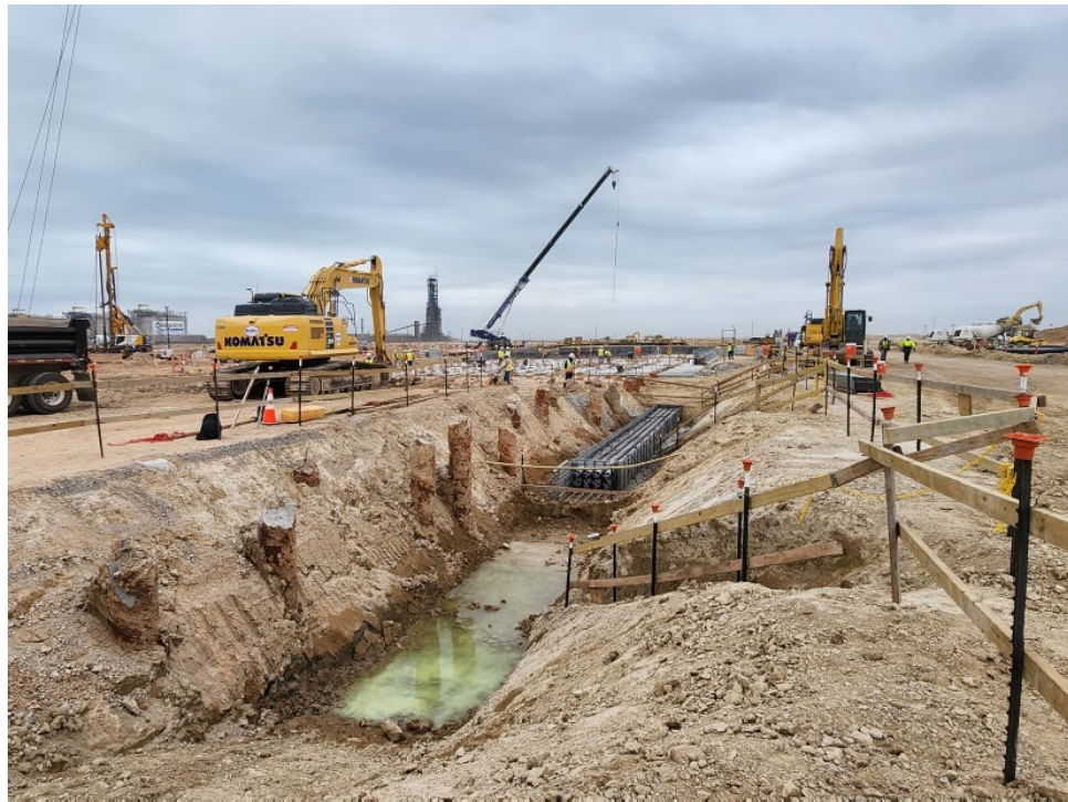
Electrical duct bank installations alongside Train 1 cryogenic area
