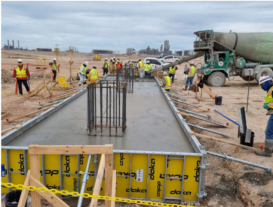
First concrete foundation poured in OSBL area
