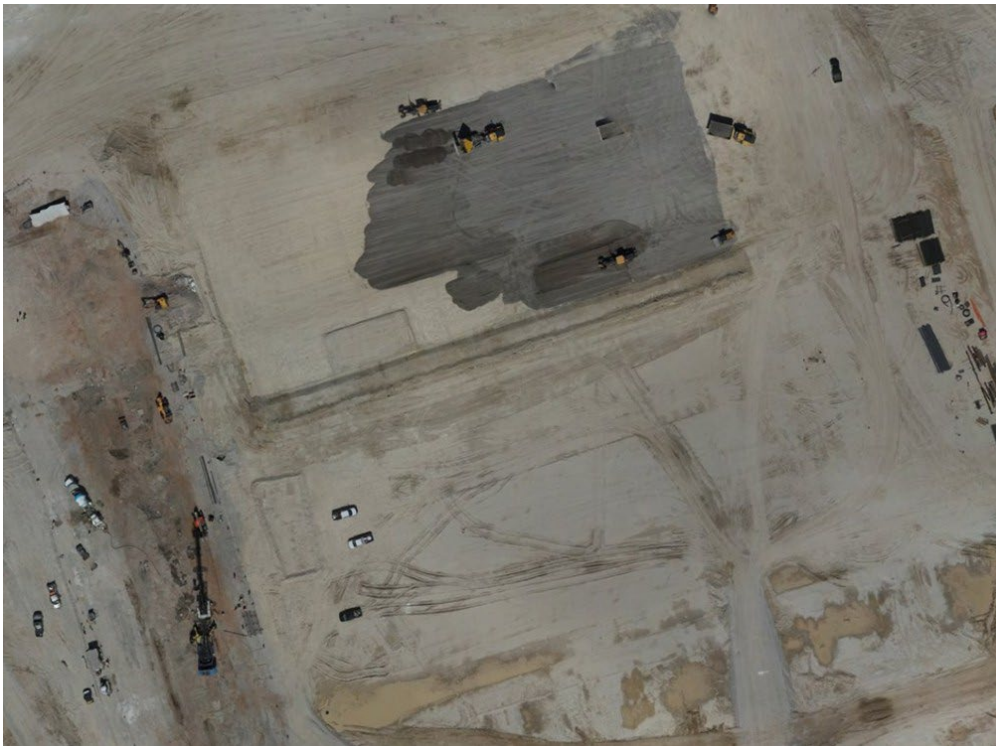
Surface preparation for piling in Train 1 footprint alongside OSBL piling installations
