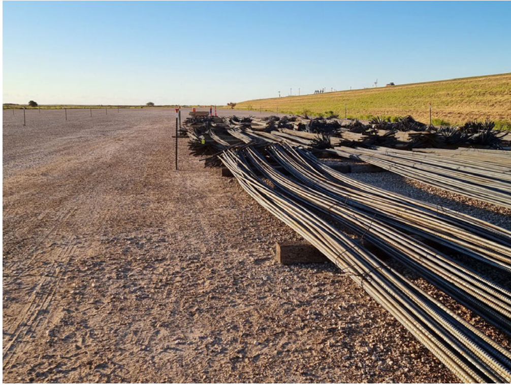
First rebar for concrete foundations
