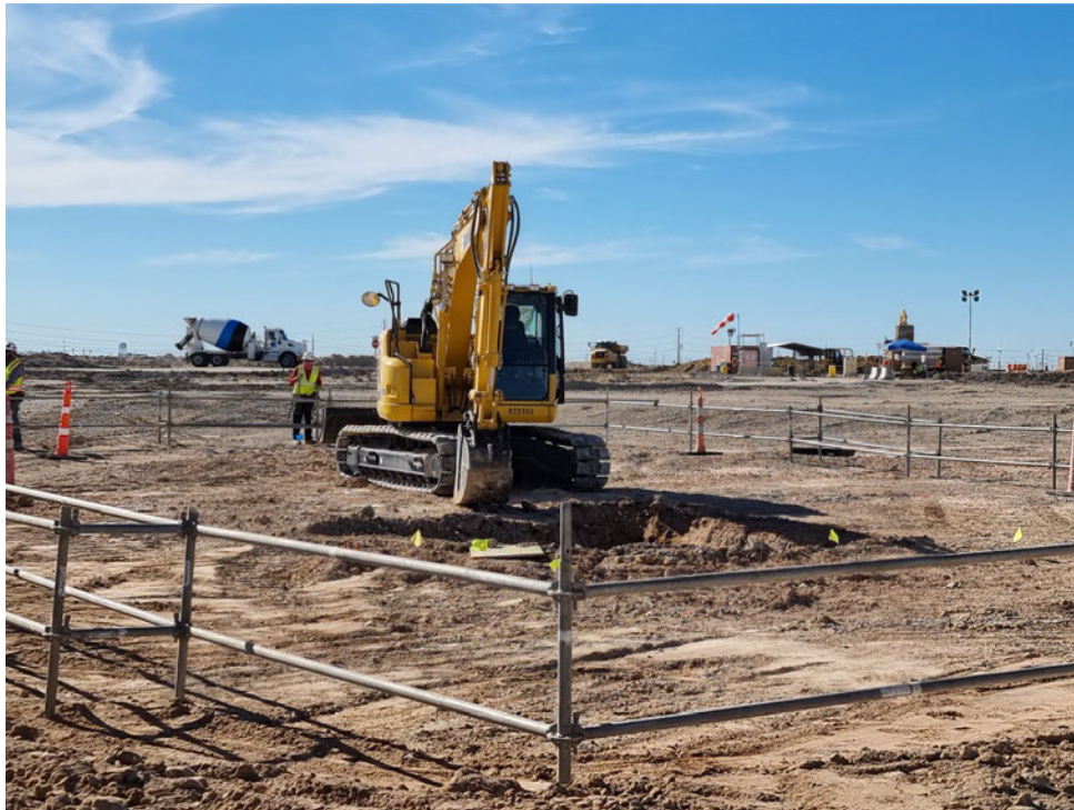
Preparation for commencement of first electrical ductbank installations
