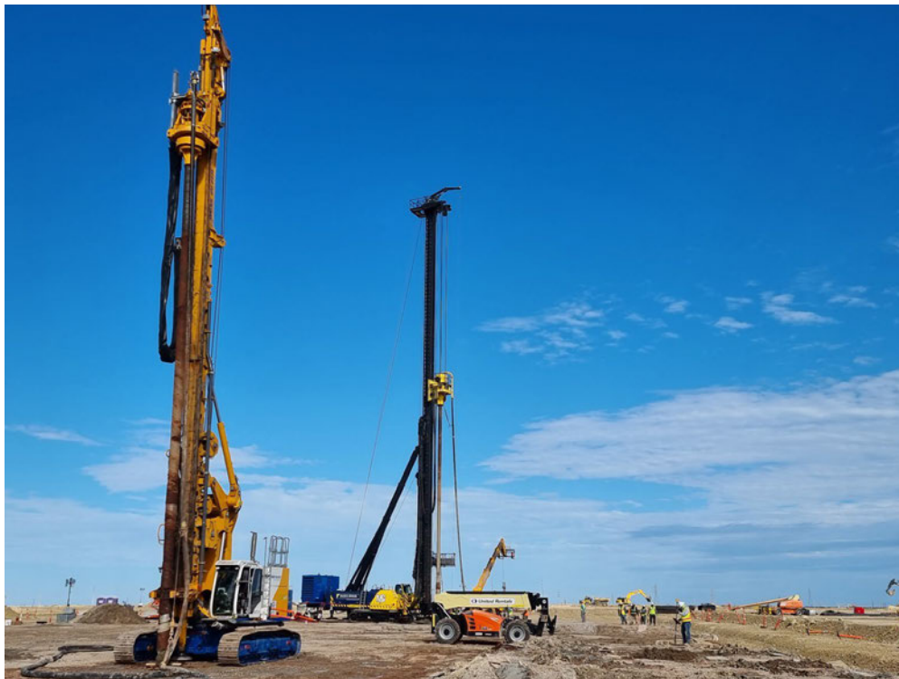
Subcontractor piling rigs in Train 1
