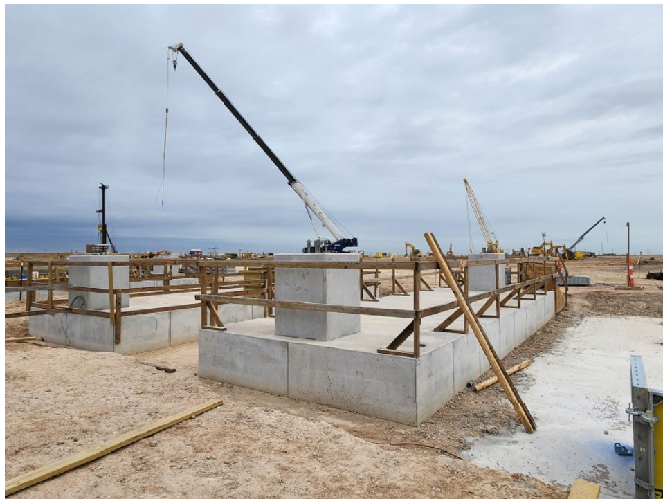
Concrete foundations and pedestals in OSBL West area
