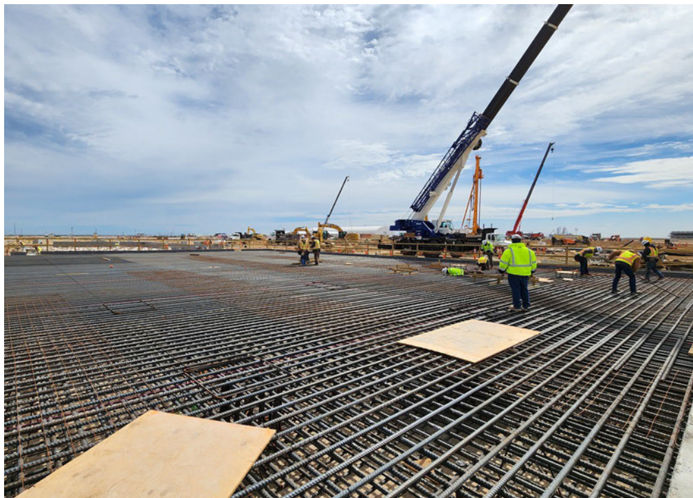
Rebar preparation for second concrete pour in Train 1 cryogenic rack area
