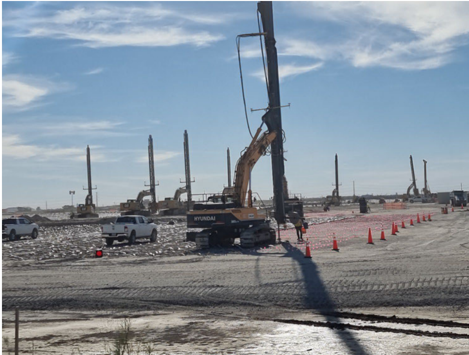
Wick drain installations
