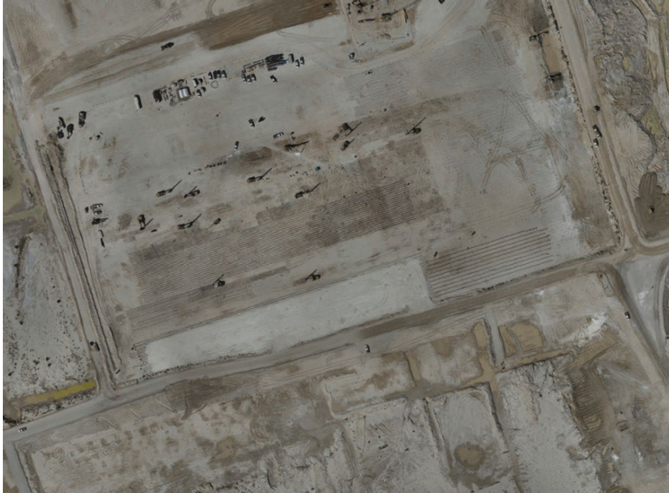
Wick drain installations in Zone 2 (Trains 4 and 5)
