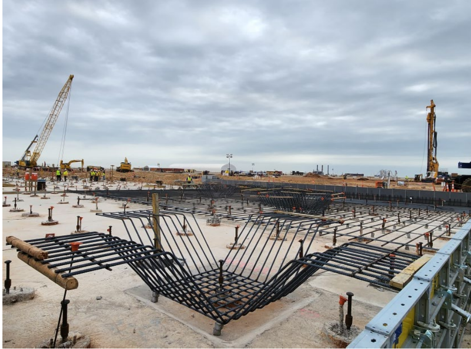
Formwork, rebar & mudmat for cryogenic rack area of Train 1
