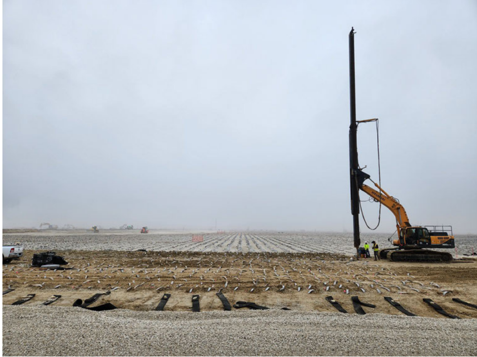
Wick drain installations progress
