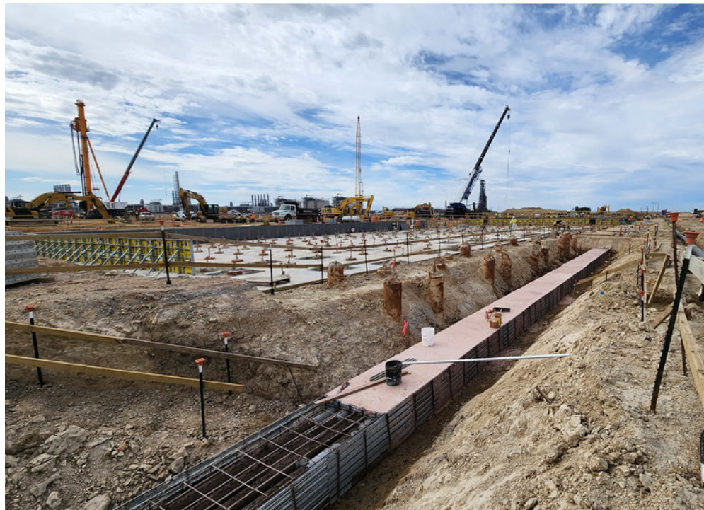
Electrical duct bank installations alongside Train 1 cryogenic rack area
