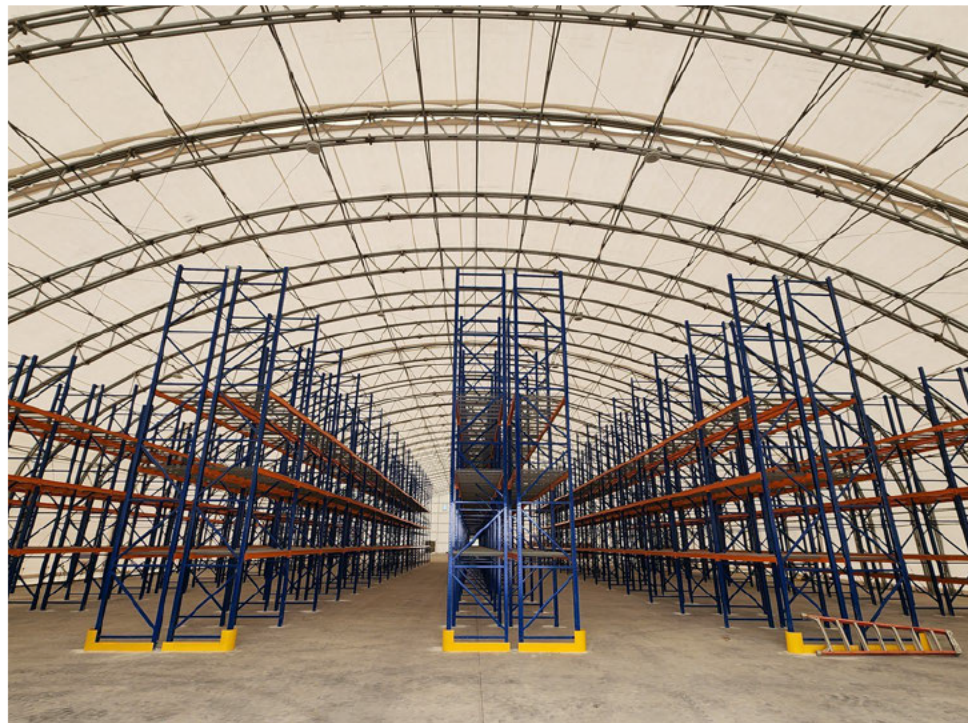
Procurement Warehouse #1 - Shelf fit-out
