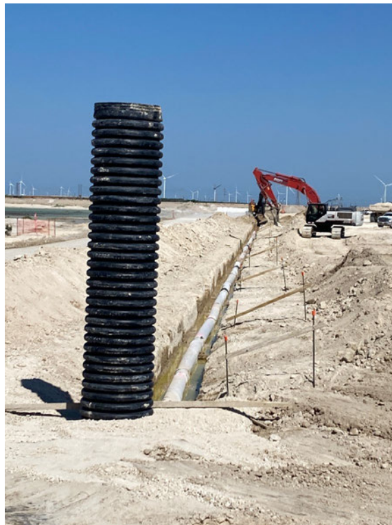
French drain installations for wick drain works
