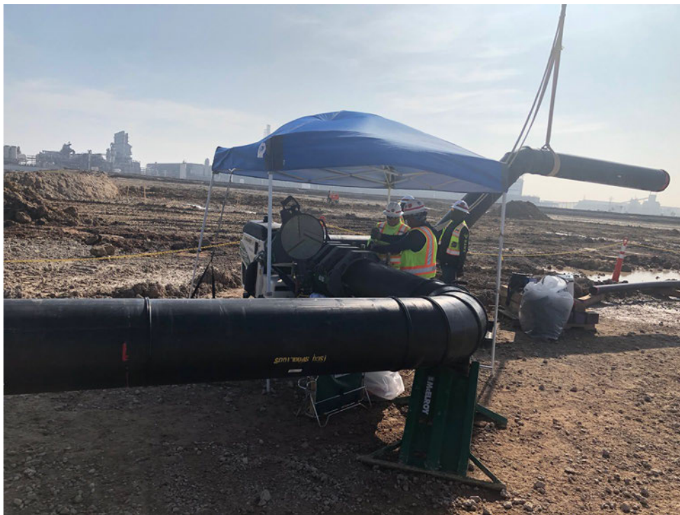
HDPE underground pipe spool prefabrication
