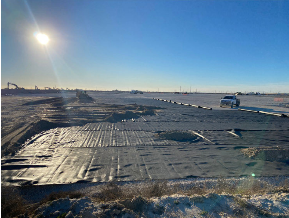
Surcharge backfill underway in Train 4
