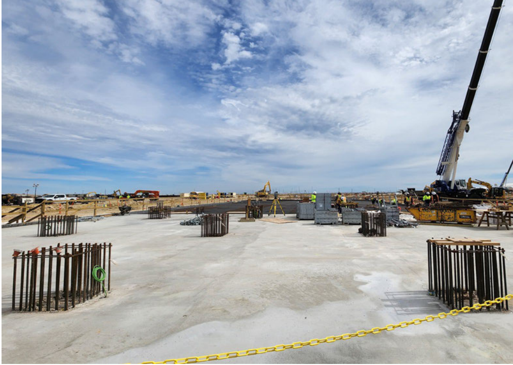
West side of cryogenic rack area 311A01- foundation and pedestals progress
