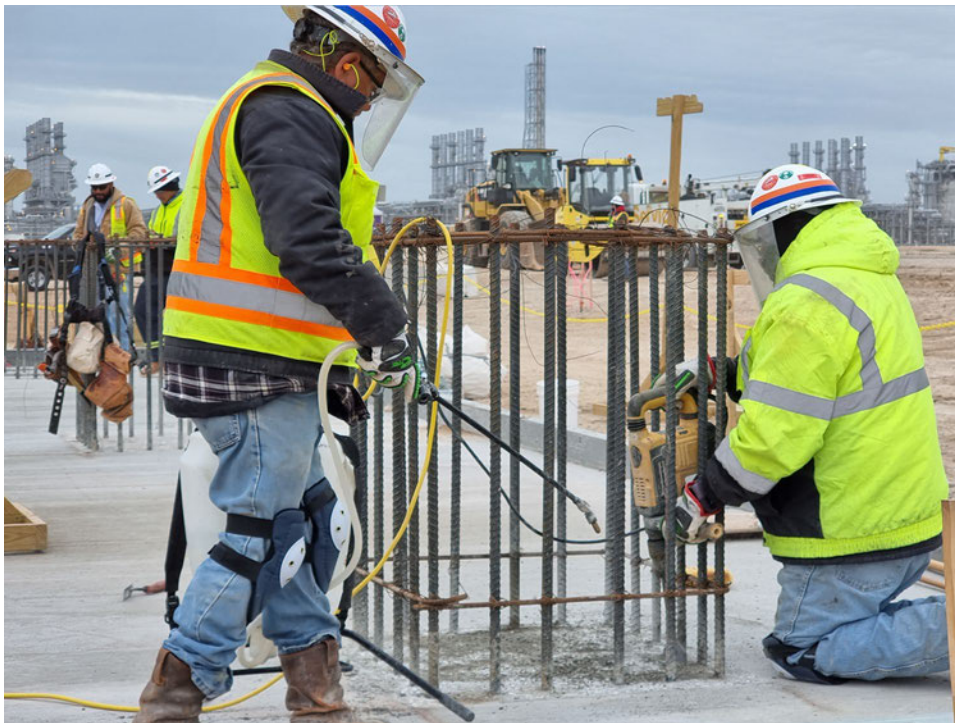
Preparation for first pedestal installations in OSBL area
