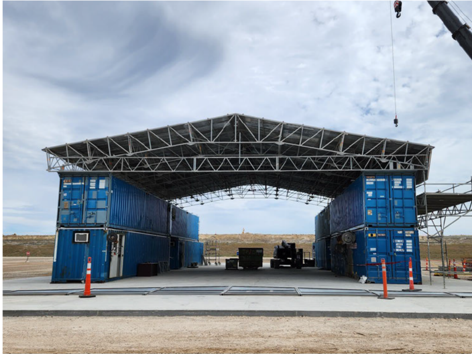
Mechanic shop installation
