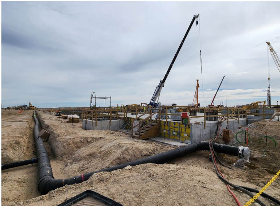
HDPE underground pipe spool installation – North of Train 1 Cryogenic rack area
