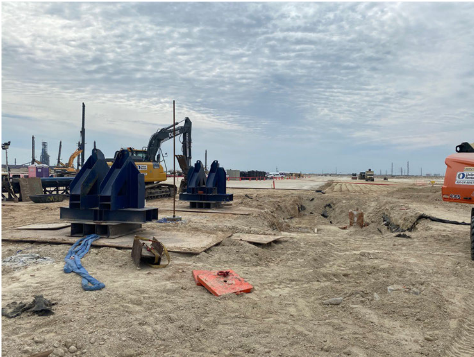
Pile load testing at Train 6 test pad
