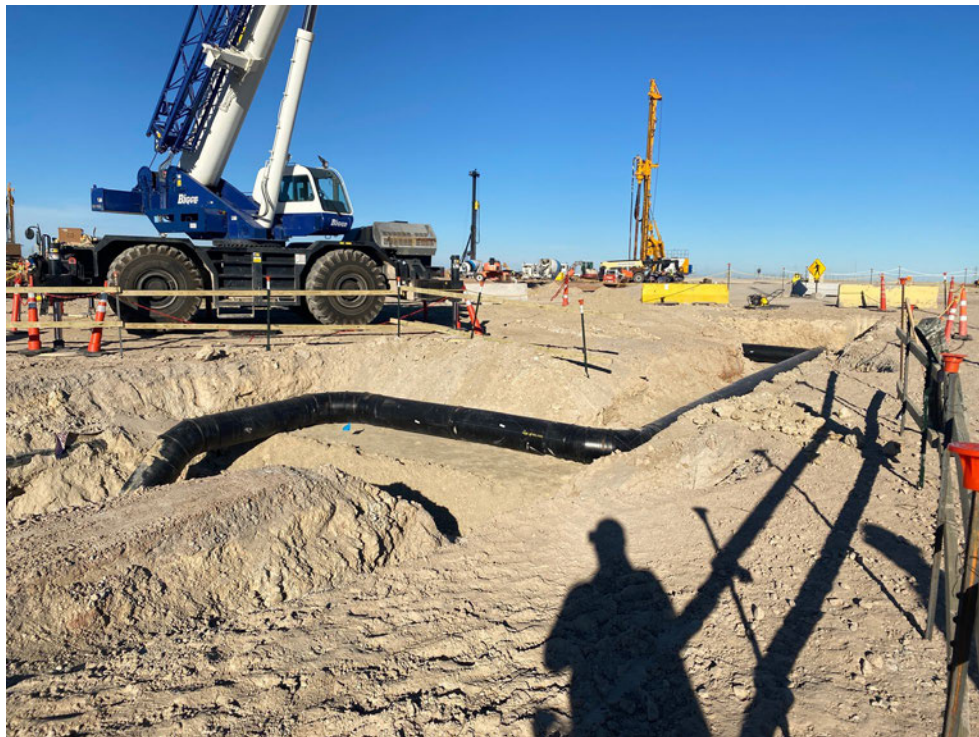
Underground firewater pipe installation
