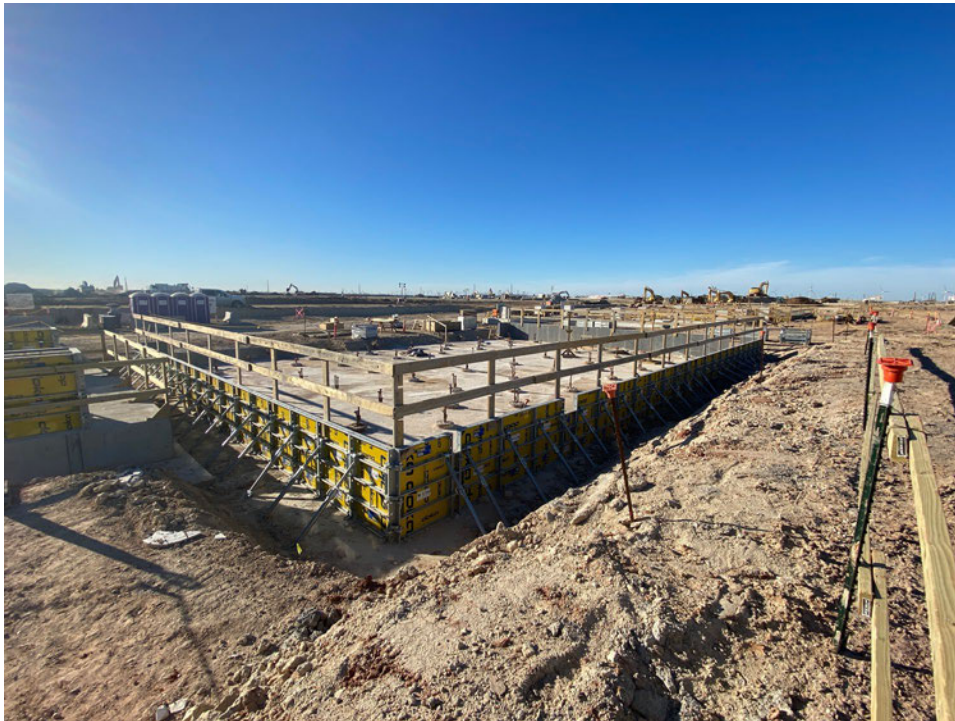
Concrete foundations and pedestals progress in OSBL area
