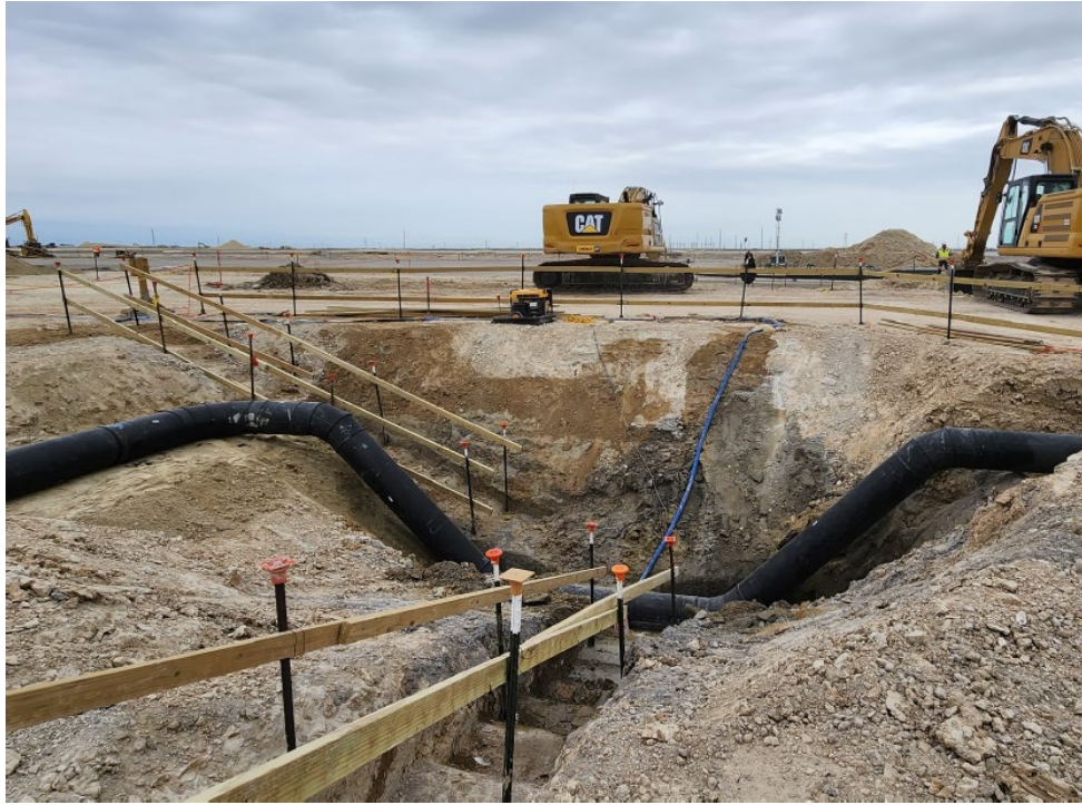
HDPE underground pipe spool installation in Train 1
