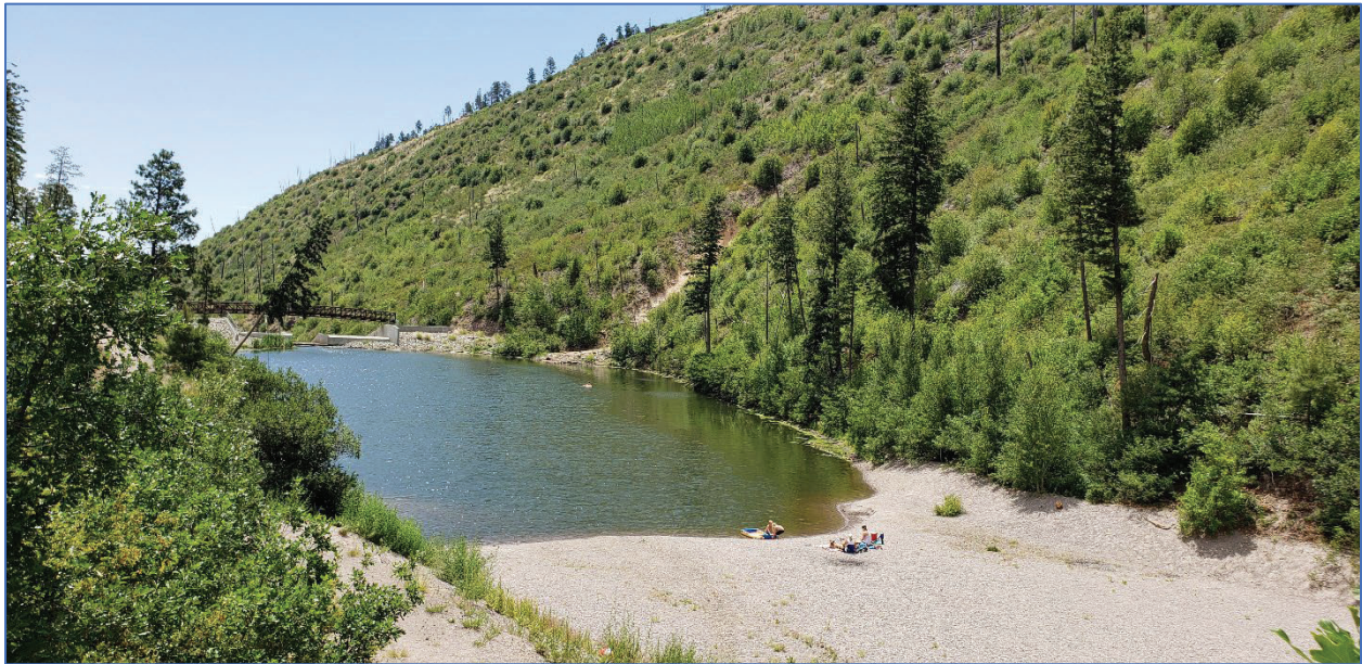
Photo 3. Sediment from the Watershed Filling the Reservoir, this sediment will be removed to increase reservoir capacity and this material will be moved downstream to create road base.
