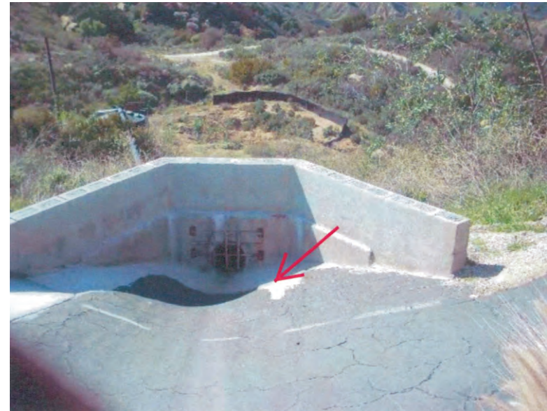
Figure 2.5f Building 4075 Subsurface Drainage to Stormwater Culvert Photograph 2009
