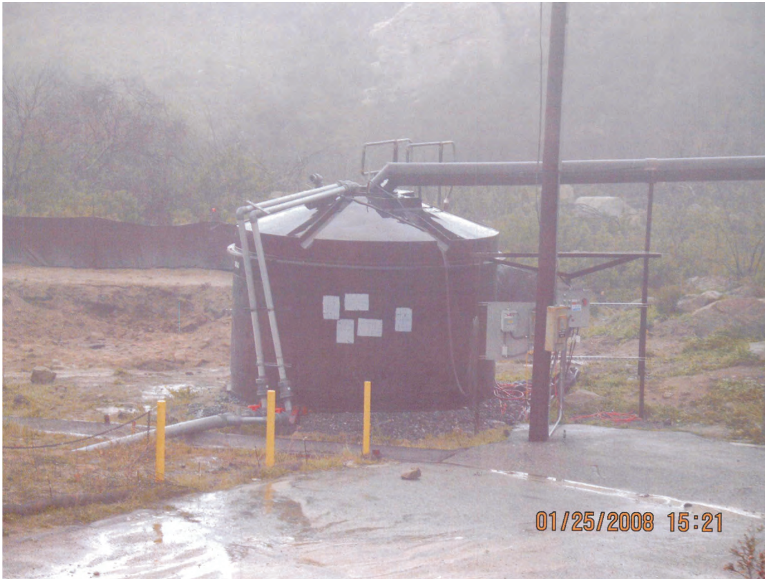
Figure 2.18f RMHF 4614 Holdup Pond Collection Tank
