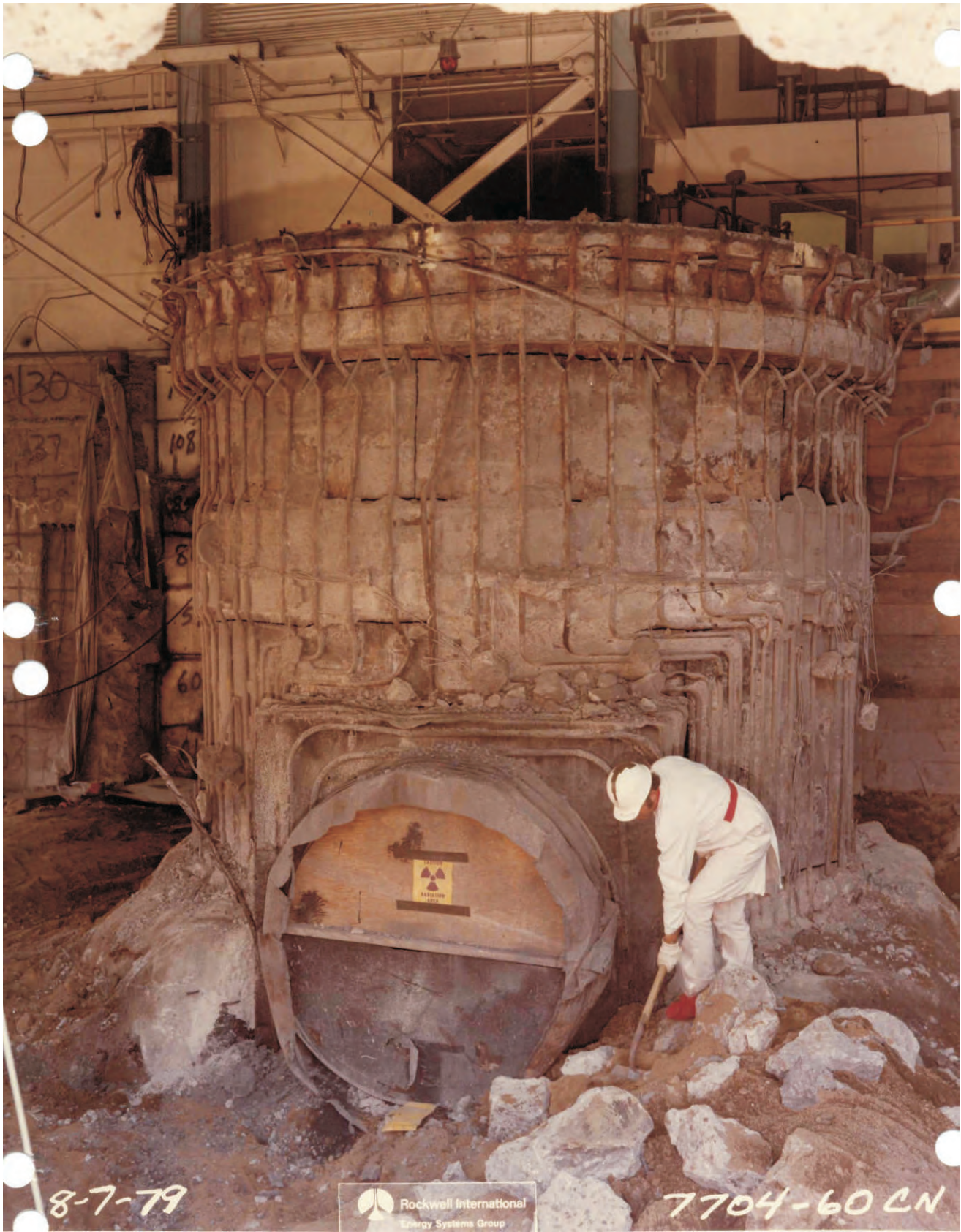
Figure 2.1.3i Building 4143 Shielding Excavation 1979
