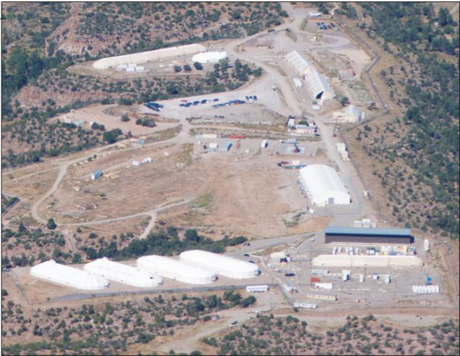
Waste Storage Domes at Area G
