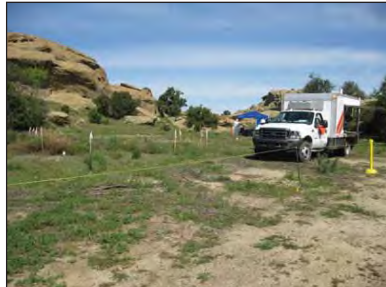
Plate 1D - Subsurface soil sampling equipment located in Subarea 5A (SS-17) in a dense stand of Santa Susana tarplant.
