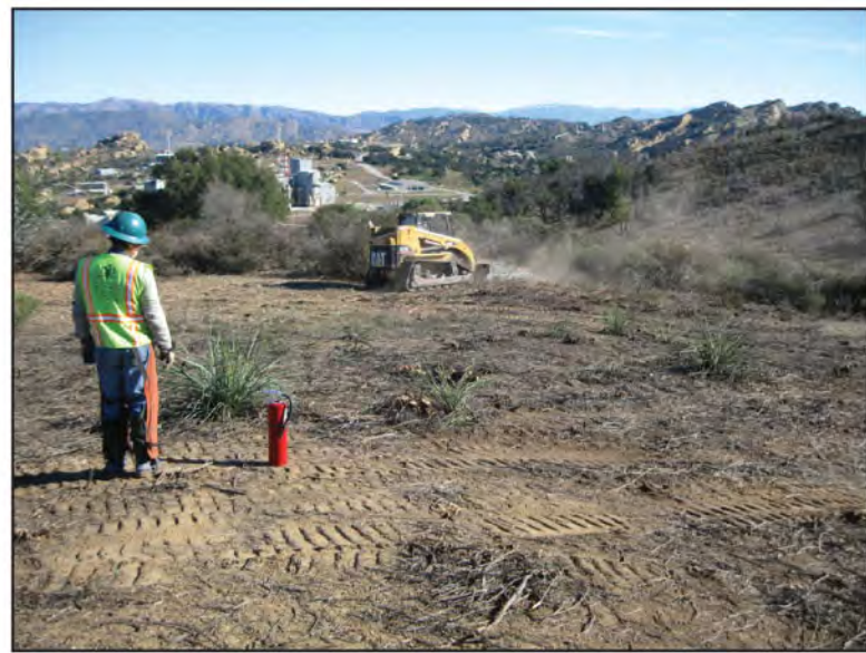
Plate 1B – Skid steer with mower attachment cutting vegetation in SS-49 (Subarea 8).
