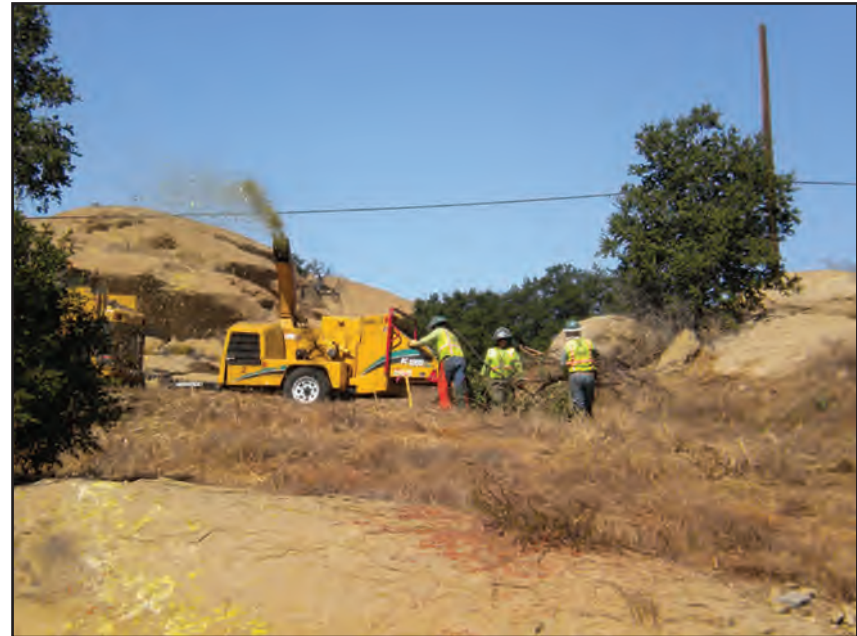
Plate 1B – Vegetation Cutting crew with chipper in SS-18.
