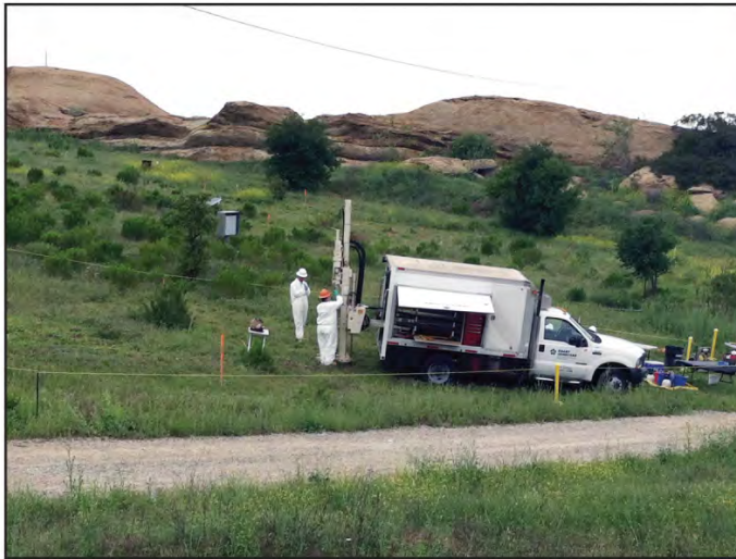
Photo 1A – Soil Sampling crew operating Direct Push Technology rig in SS-46. Photo taken May 2, 2012.
