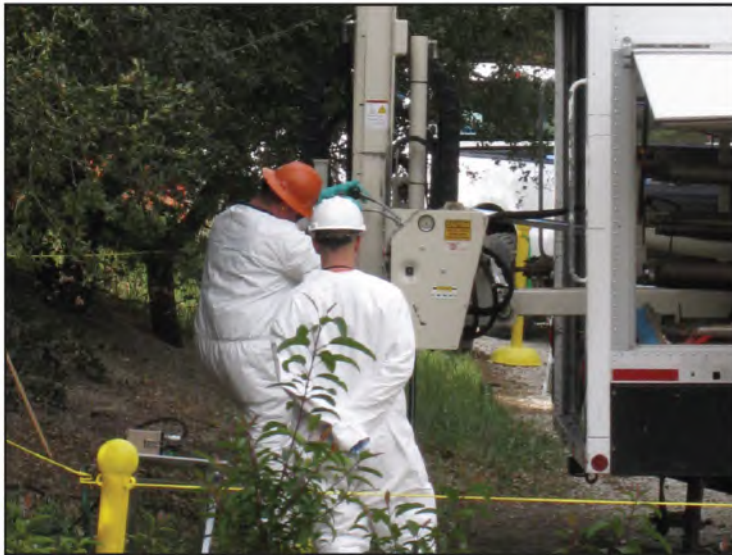
Plate 2A – Soil sampling activity using a Geoprobe Direct Push Technology (DPT) rig in Subarea 5C while avoiding impacts to protected trees. March 5, 2012.
