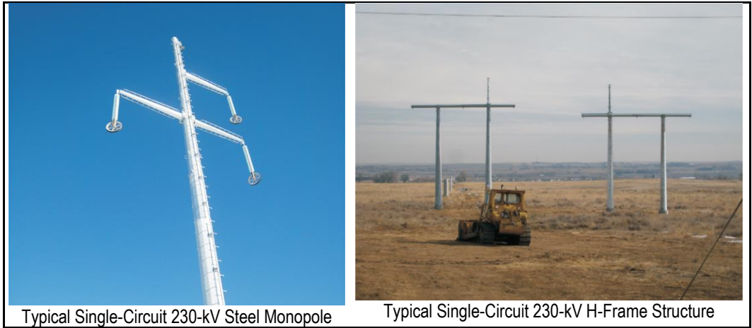
Figure 2-2 Typical Transmission Line Structures
