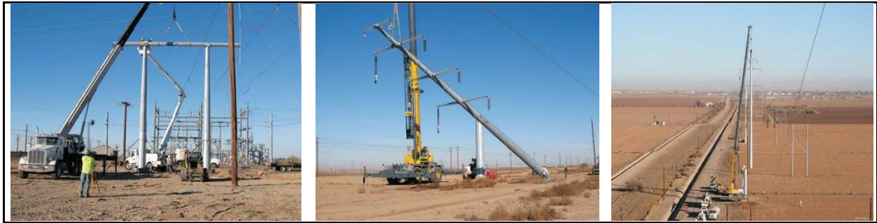
Figure 2-5 Typical Construction of Transmission Line Structures
