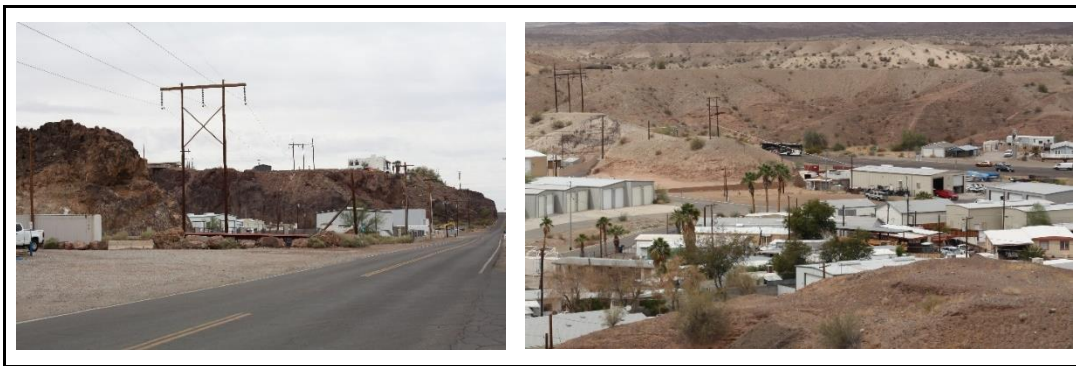
Figure 1-2 Examples of Encroachment onto WAPA's Right-of-Way
