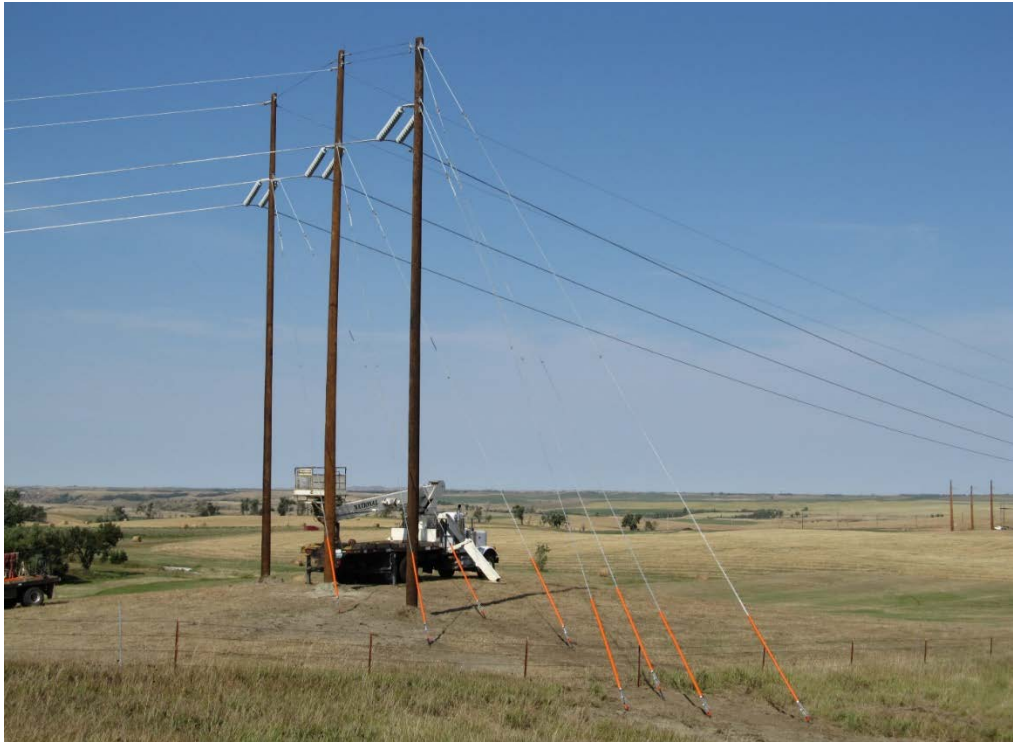
Photo 1: Guy wire installation
