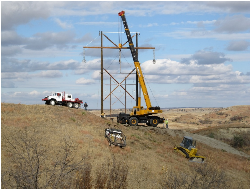
Photo 3: Grading at a structure site to level crane set-up.
