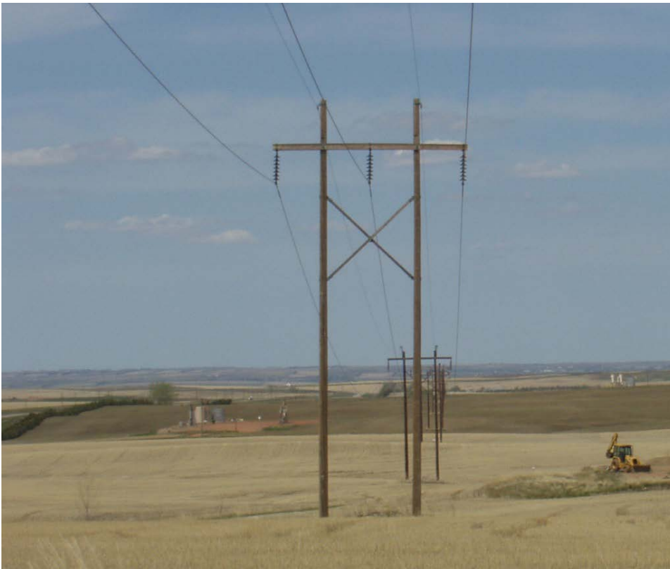
Photo 4: The structure in the foreground is an example of the structure design that WAPA is proposing to install. The structures in the background are the original structures, which WAPA is proposing to replace.
