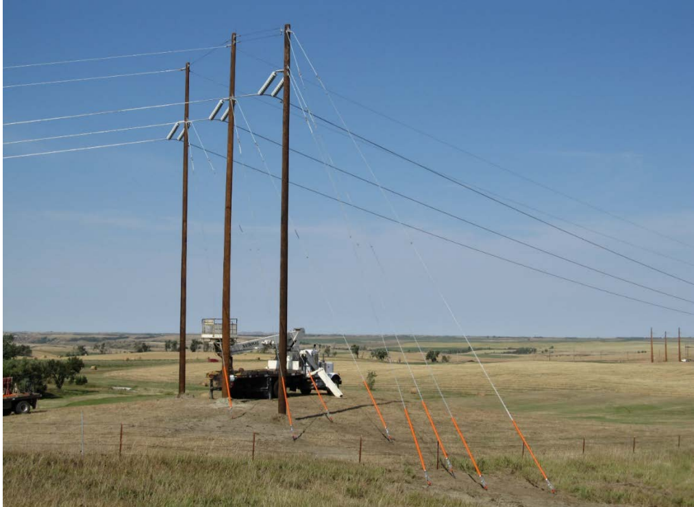
Photo 1: Guy wire installation
