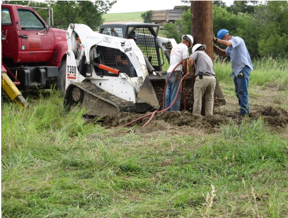
Photo 5: Typical earth disturbance at pole locations during hole auguring.
