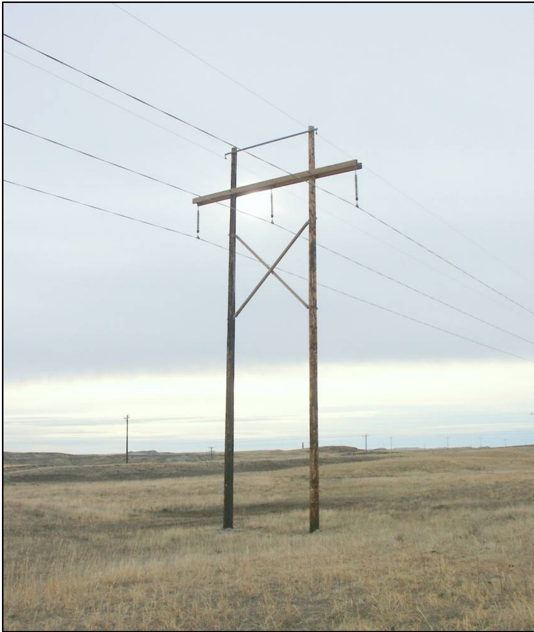
FIGURE 2.3-2 STANDARD H-FRAME 115-KV STRUCTURE
