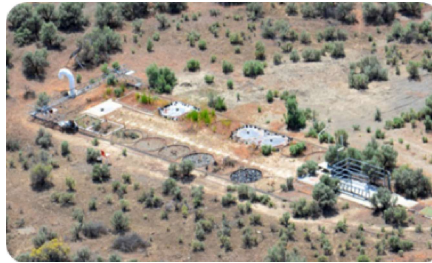
Aerial view of Lysimeter Location
