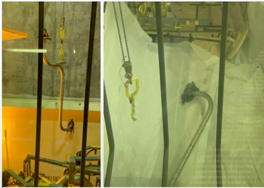
Jumper Removal and Stage for Bending
