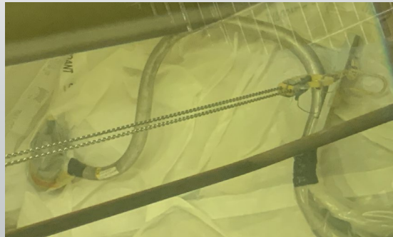
Jumper Bending Completed
