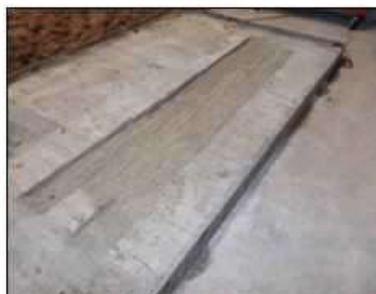
3 Passes on 7:1 Mix Concrete
