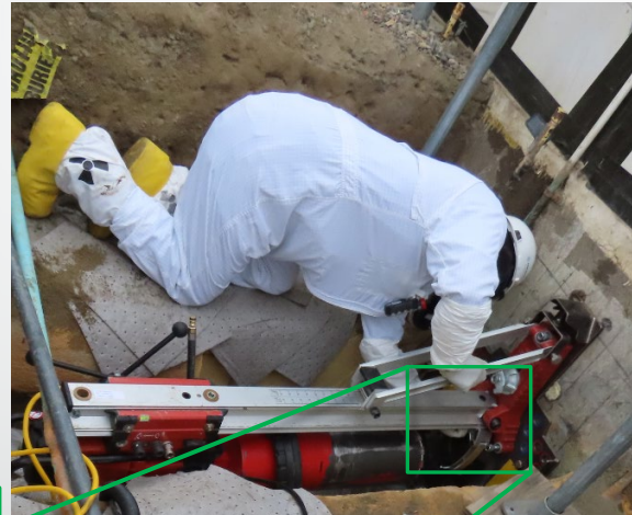
Installation of Drill Guide and Core Drill
