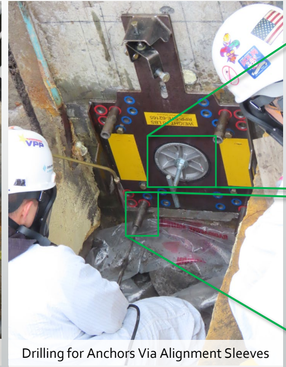
Installation of Drill Guide and Core Drill
