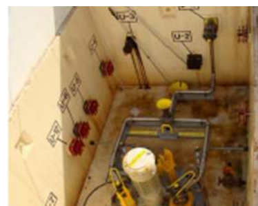
Typical Central Pump Pit
