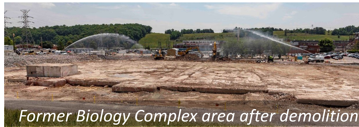
Biology Complex demolition
