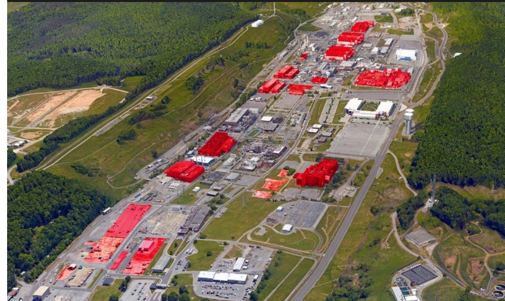
Facilities to address at Y-12
