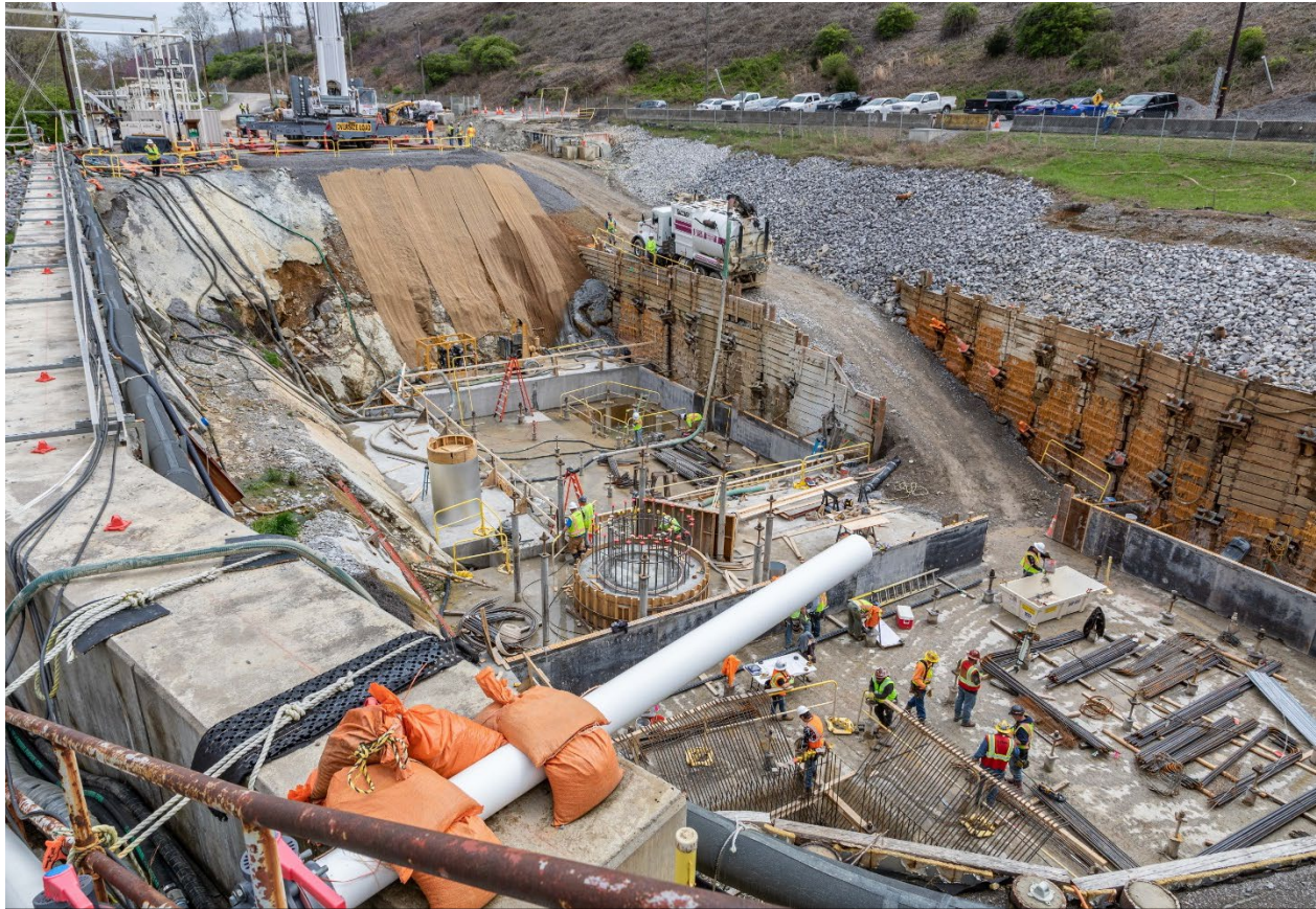
Construction on MTF headworks facility
