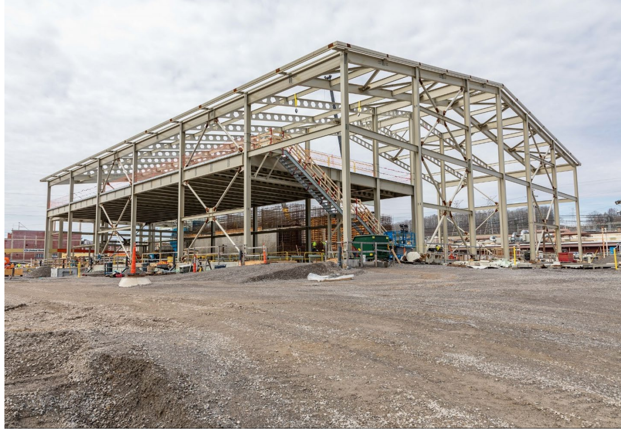
Construction on MTF treatment facility
